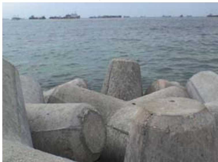
Tetrapod seawall around Male’
