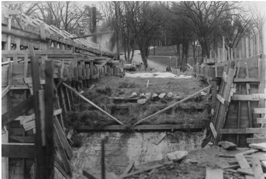
Laying the 24-foot road. Note old wooden structure at left.
