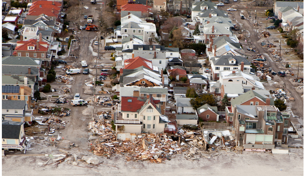
Hurricane Sandy damage, Long Beach, NY. Credit: Andrea Booher, FEMA
