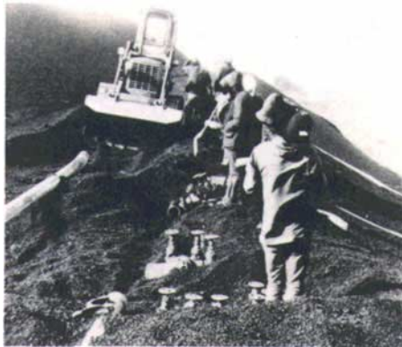
On May 4, 1973, workmen laid additional pipes to carry seawater up onto the lava flow front and tephra bulwark to cool and harden the still-flowing lava behind the chilled lava margin.
