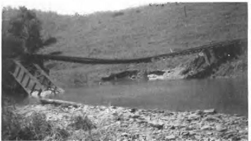
FIGURE 4.—Washed-out railroad bridge on Copen Run. Courtesy of Corps of Engineers.
