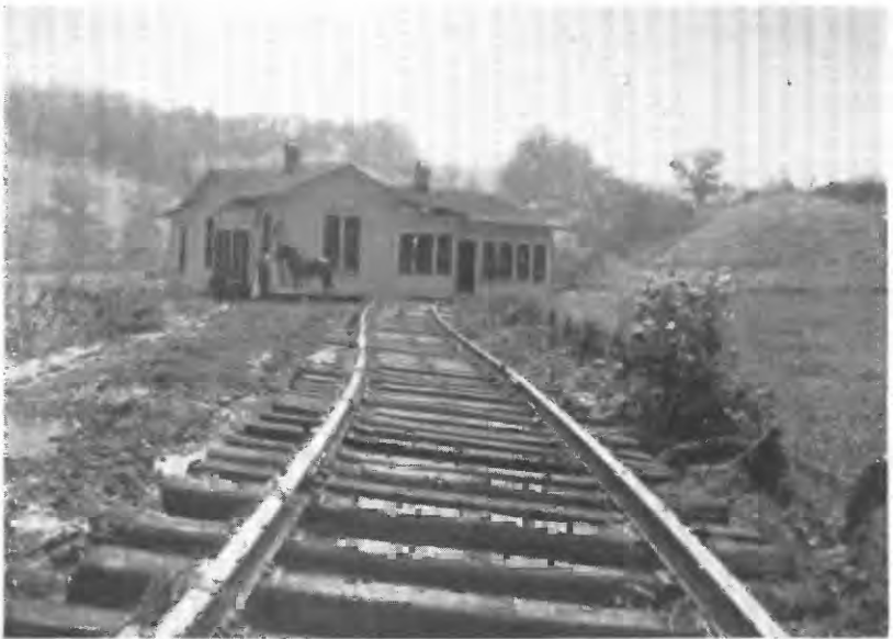
FIGURE 3.—Residence near Heaters, which with its four occupants was washed a mile down O'Brien Fork of Saltlick Creek and lodged on a displaced section of railroad track. Courtesy of Baltimore & Ohio Railroad Co
