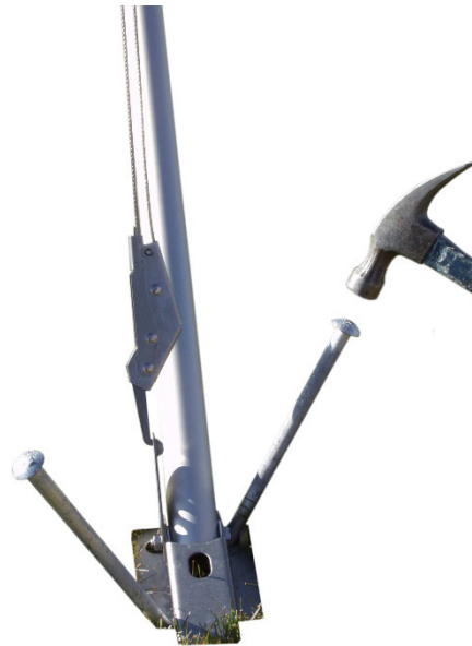
FIGURE 6-11. Staking the tripod feet
