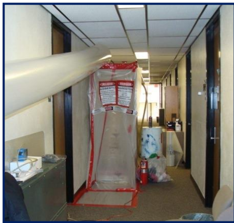
Figure 21: Asbestos Abatement
