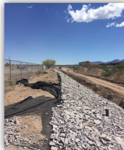
Figure 28: Storm water Inspection
