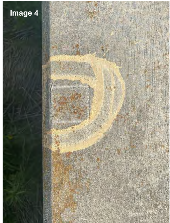
Image 3: North Carolina DOT benchmark with RTN placed vertically above the BM. Note the DOT metal disc has yellow paint around it to help identify it more easily.
