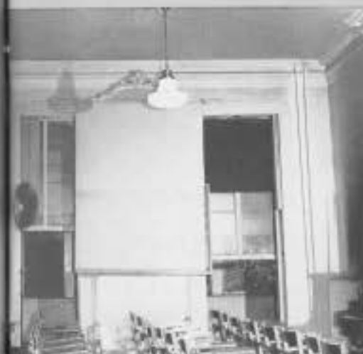
Above—Classroom at the American University before modernization.
