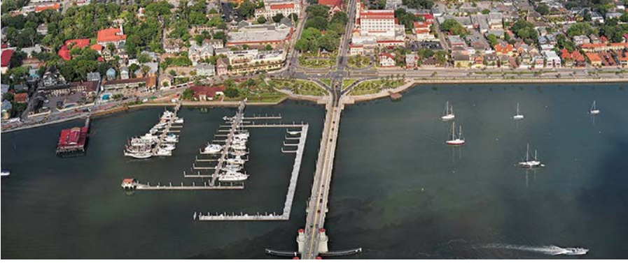
Historic St. Augustine is one of many communities along the Florida coast subject to flooding due to rising sea levels.
