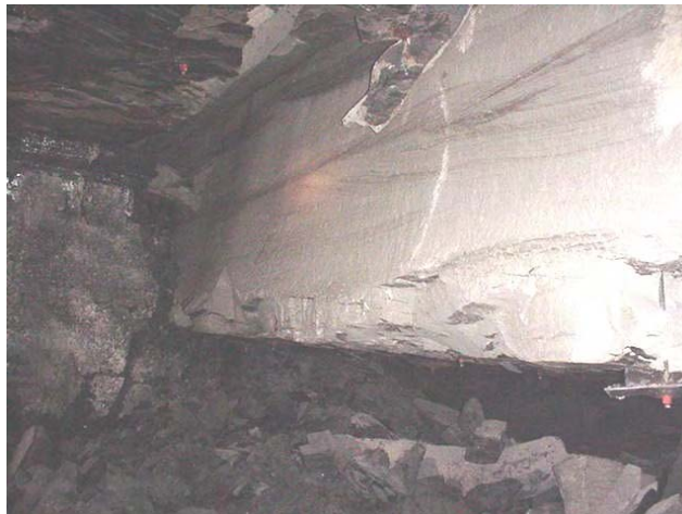
Figure 8.—Damage caused when open entries were subsided.
