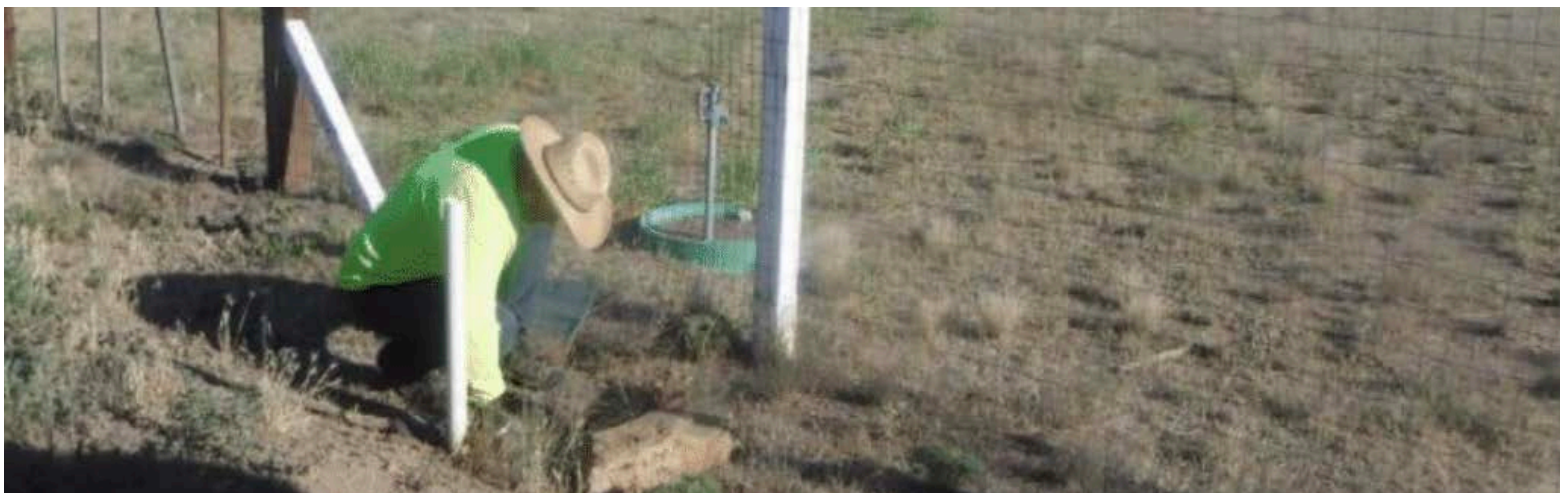
Contractor installs an acoustic leak detection sensor
