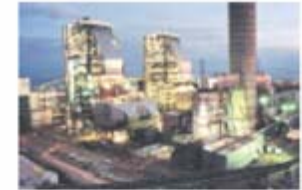
Similar Power Plant
