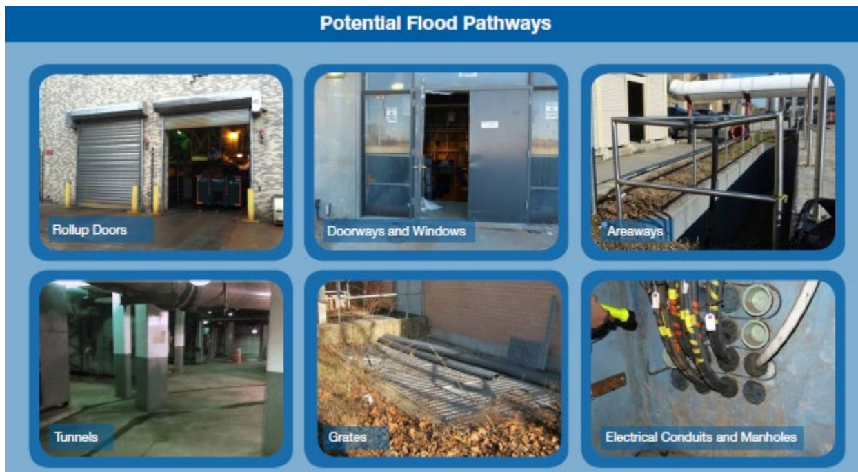
Figure 1. Common flood pathway examples from the New York City Wastewater Resiliency Plan (2013).
