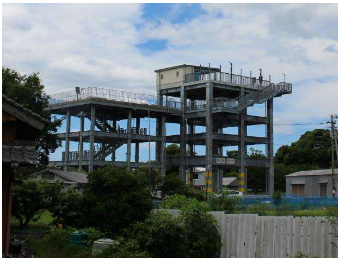
Construction of the tower (Local gov't)
