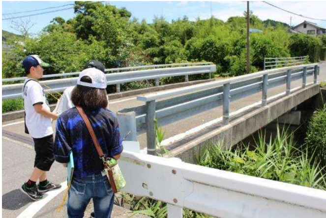
Retrofitting of the bridge over evacuation route
