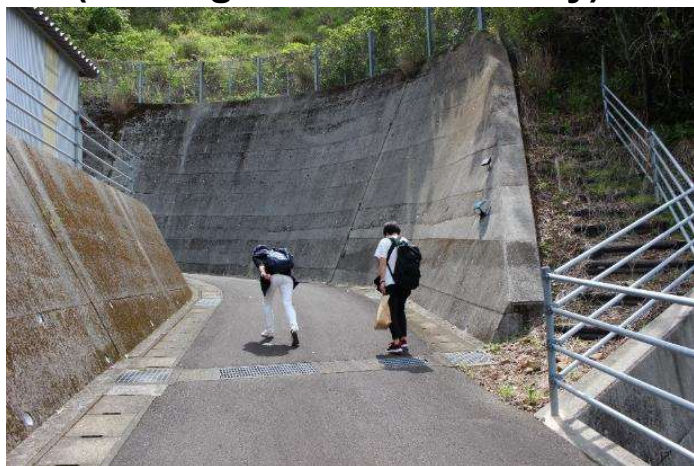
Construction of evacuation routes (Local gov't)
