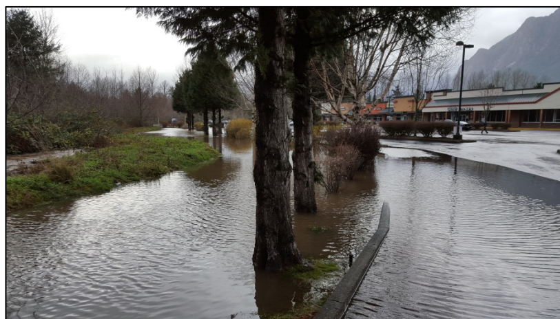
Flooding on commercial parking lots built along Ribary creek in North Bend, WA. Photo credit Jonathon Loos.
