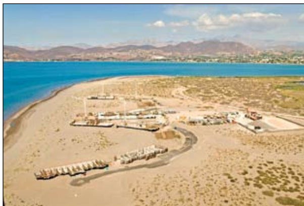
Marina construction, Paraíso del Mar.
