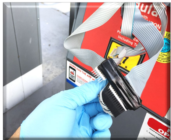
Photo 33: Internal Skimmer Found Inside a Fuel Dispenser Cabinet
