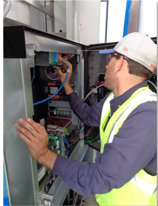
Registered Service Agent Making Repairs
