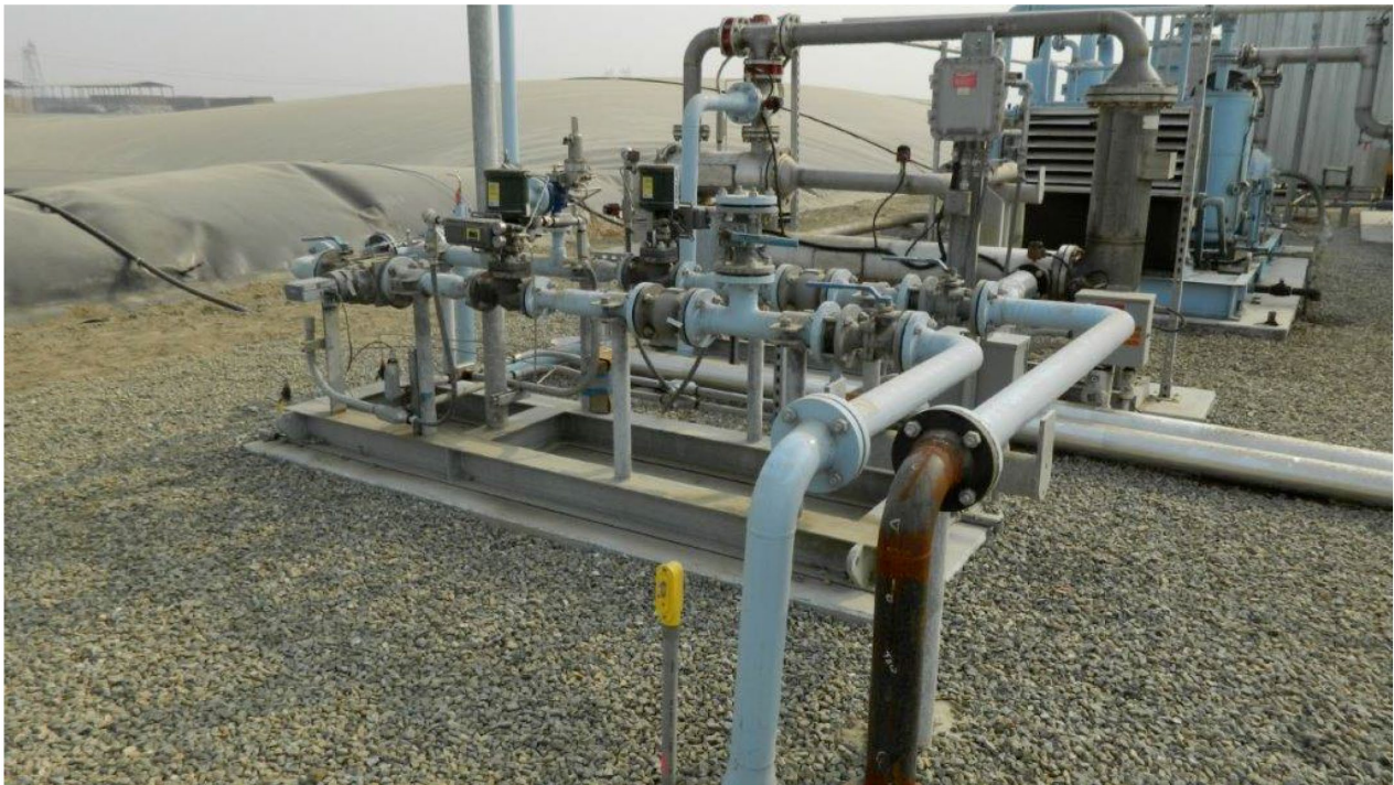
Image 20. Gathering line array (foreground) and covered lagoon digester (background) at T&W Dairy.
