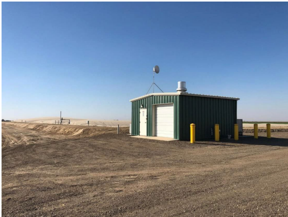
Image 8. View of biogas handling building (foreground) and covered lagoon digester (background) at Circle A Dairy.
