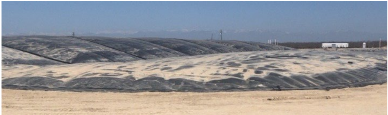
Image 36. Biogas build up in the new covered lagoon digester at Horizon Jerseys Dairy.
