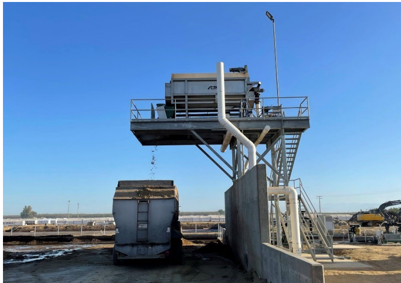
Image 39. Solid separator at Mellema Dairy.
