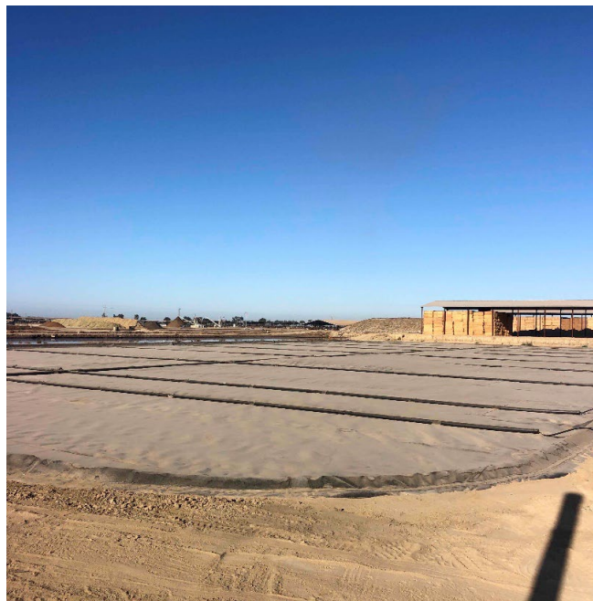
Image 26. Covered lagoon digester at Hamstra Dairy.
