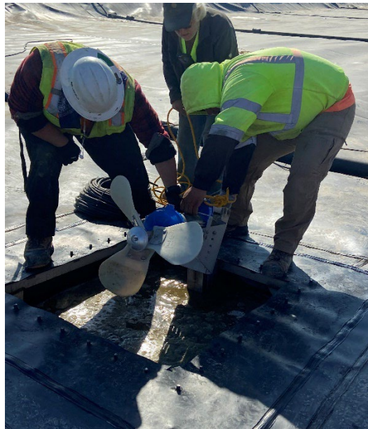
Image 31. Installation of a mixer in the covered lagoon digester at Lone Oak#1 Dairy.
