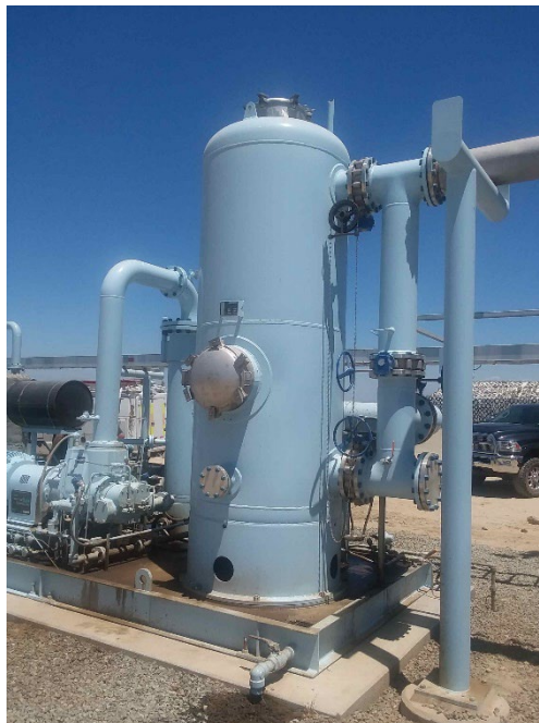
Image 32. Activated Carbon Vessel at Double J Dairy.
