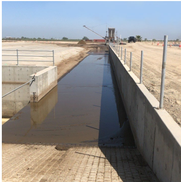
Image 49. New sand lane at El Monte Dairy.
