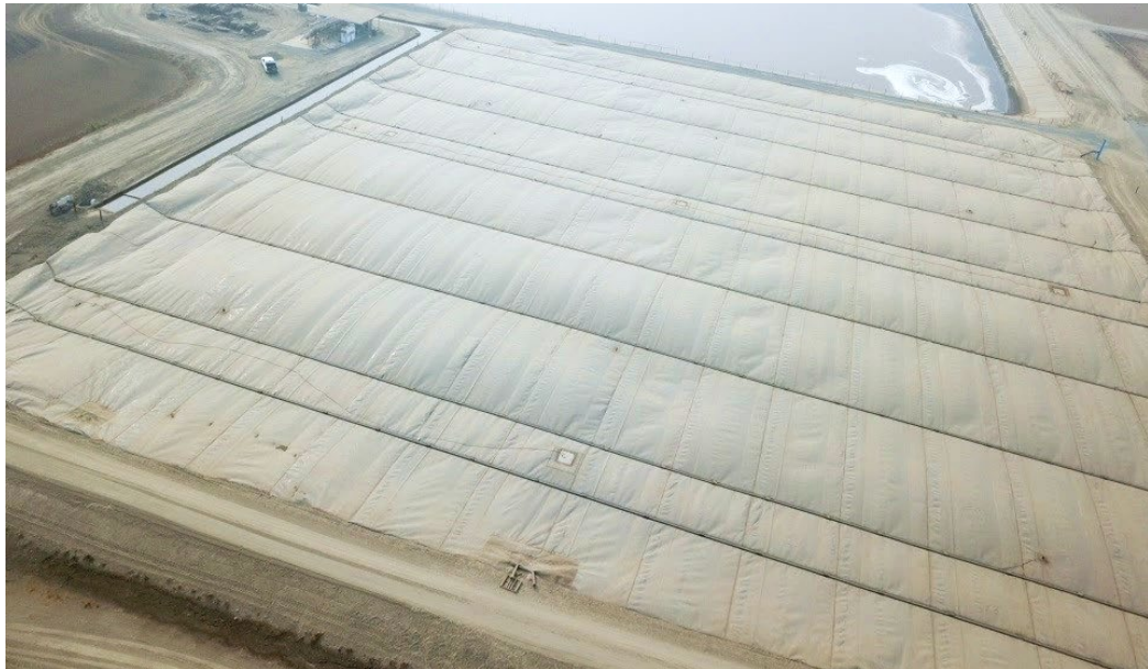
Image 51. New covered lagoon digester at Decade Dairy.
