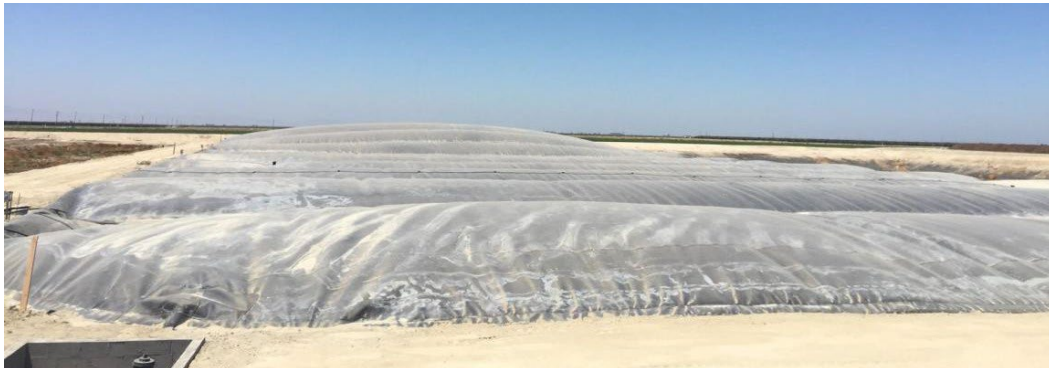
Image 3. Covered lagoon digester at Verwey-Madera Dairy.
