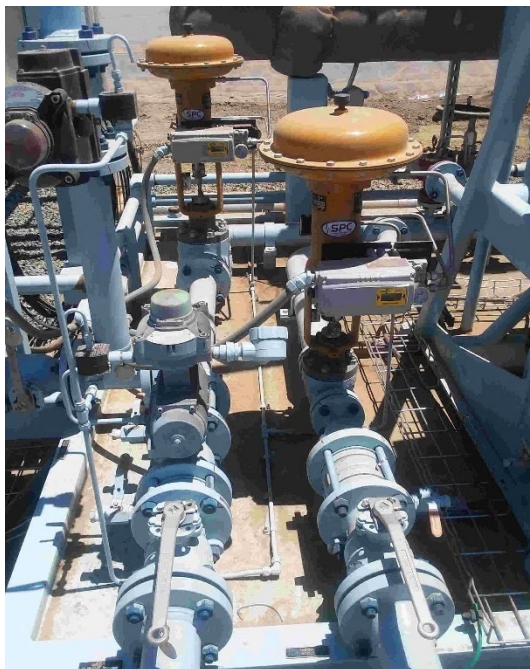
Image 38. Metering equipment at Mineral King Dairy.
