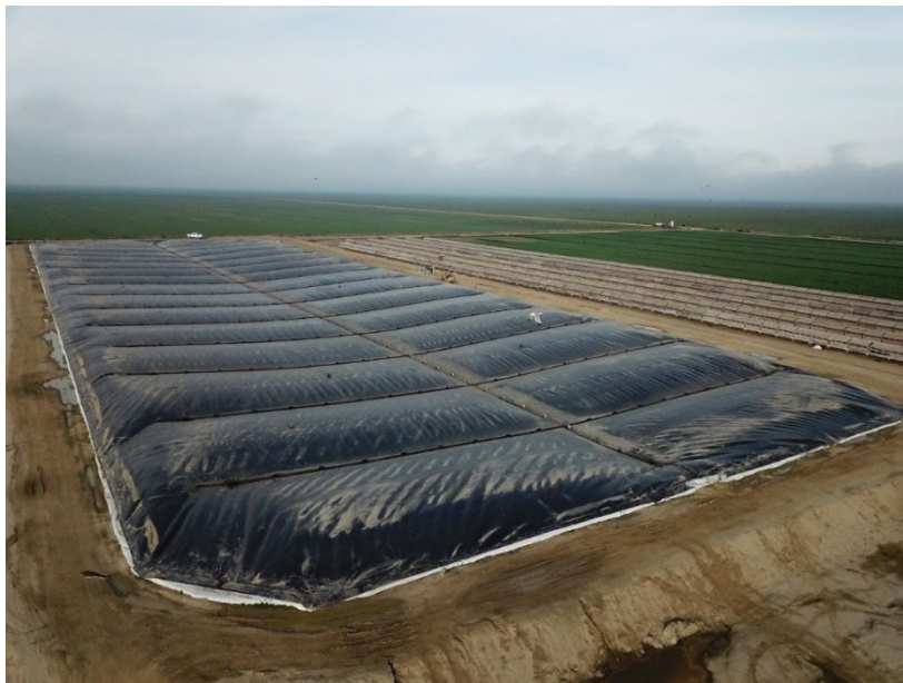
Image 16. Aerial view of the covered lagoon digester at 4K Dairy.
