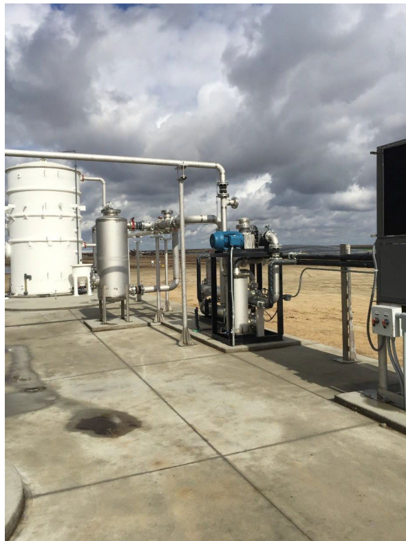
Image 5. Biogas conditioning and electric generation equipment (foreground) with covered lagoon digester (background) at the West-Star North Dairy.
