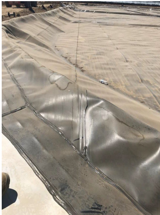
Image 14. Details of the digester lagoon cover at K&M Visser Dairy showing welded liners to prevent biogas leakage.
