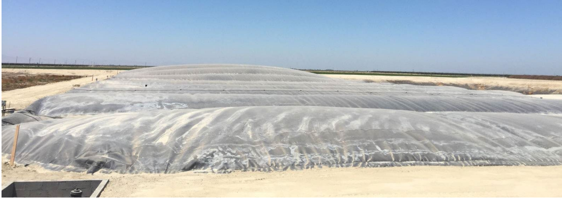
Image 5. Covered lagoon digester at Verwey-Madera Dairy.
