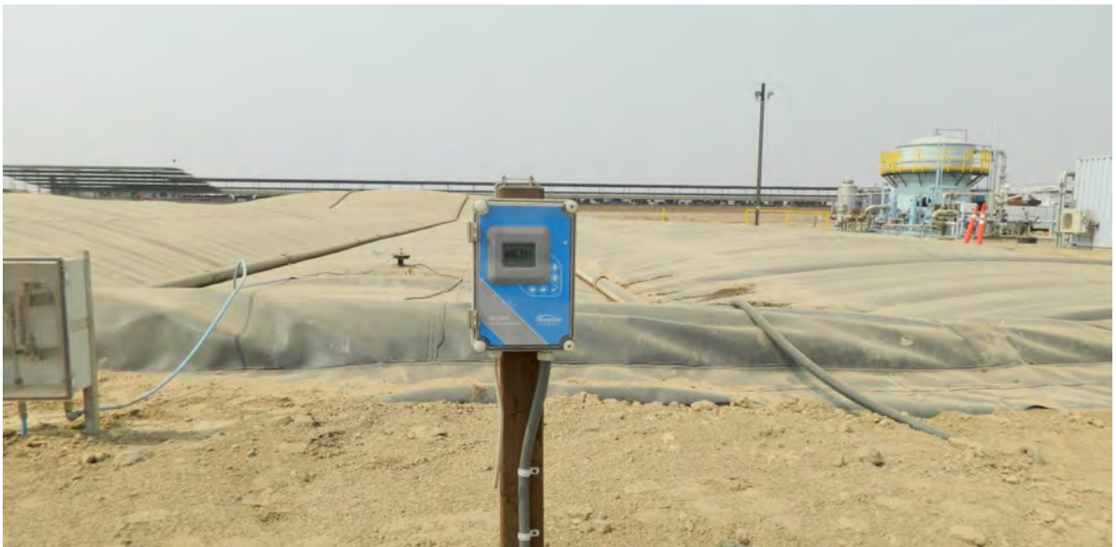
Image 18. Weir box and a weir box meter (foreground) and covered lagoon digester and biogas conditioning equipment (background) at Maple Dairy.
