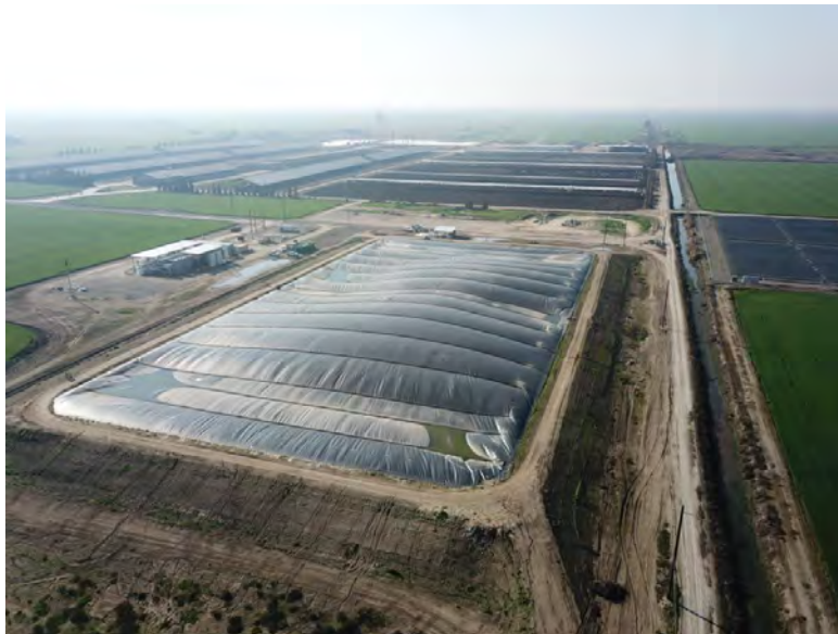
Image 62. New covered lagoon digester at Vander Woude Dairy.
