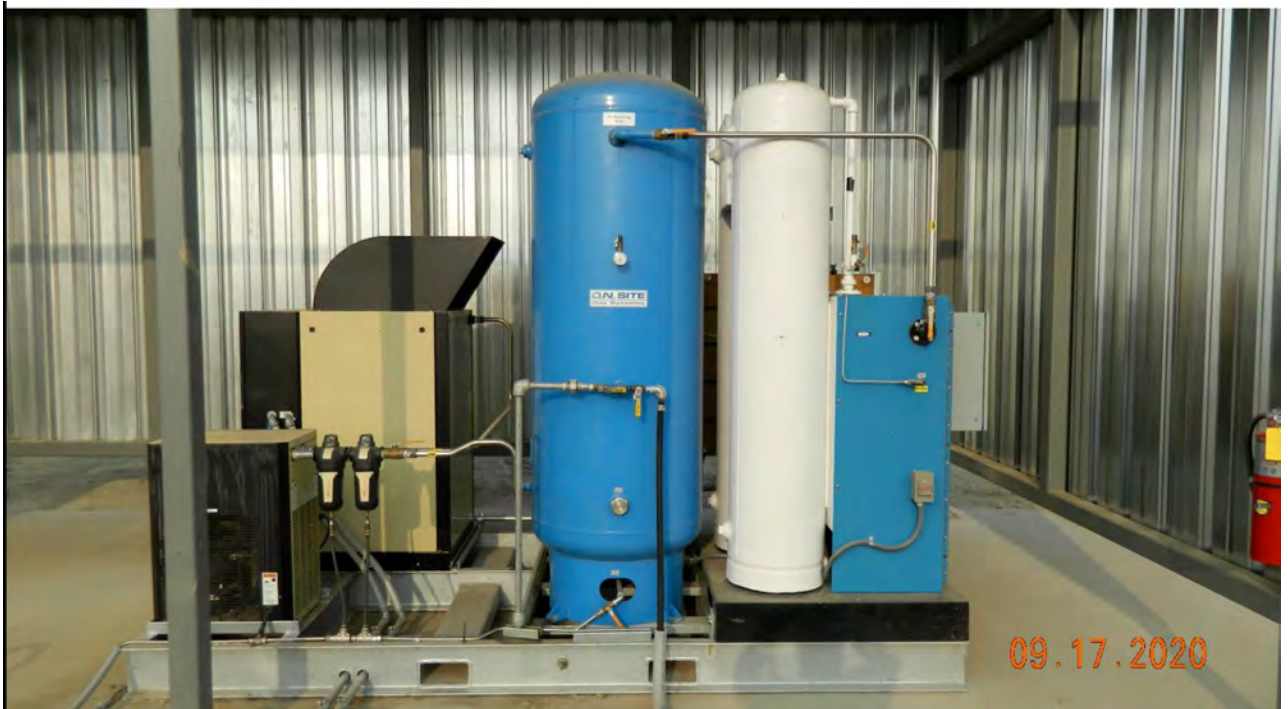
Image 19. An oxygen generator skid for biological control of hydrogen sulfide (H 2 S) at Trilogy Dairy.
