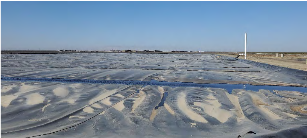
Image 70. New covered lagoon digester at Vanderham Dairy.
