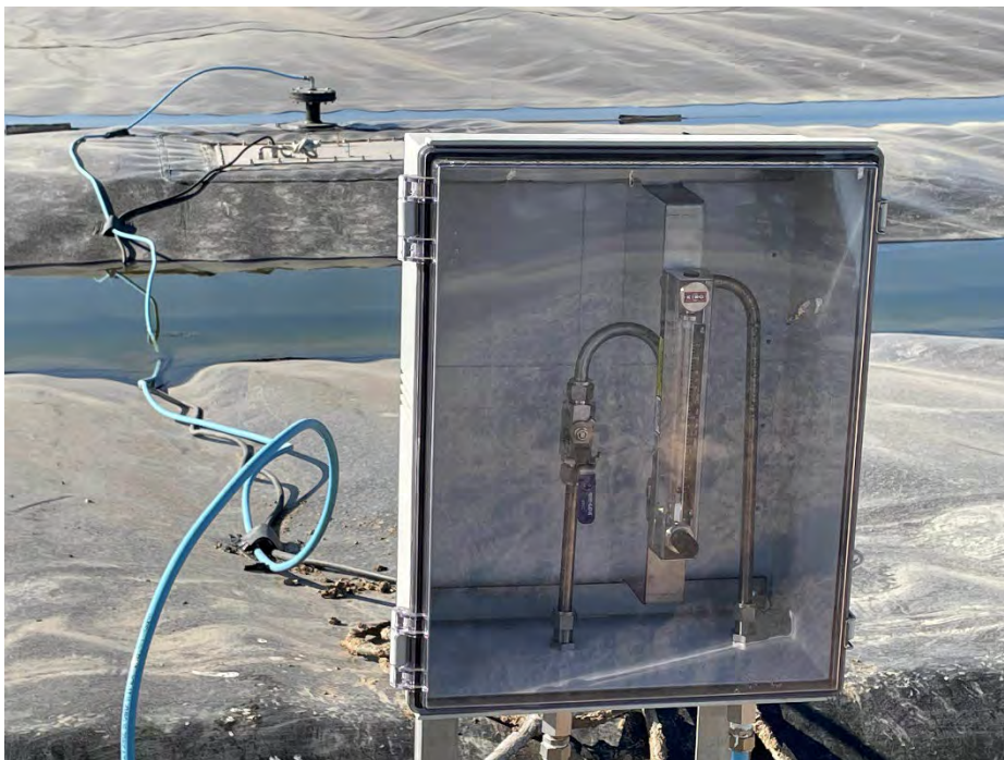
Image 71. Oxygen rotameter and oxygen injection port at Elk Creek Dairy.
