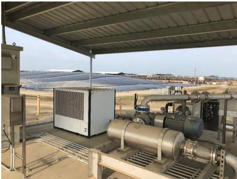
Image 15. Biogas conditioning equipment (foreground) and covered lagoon digester (background) at Riverview Dairy.
