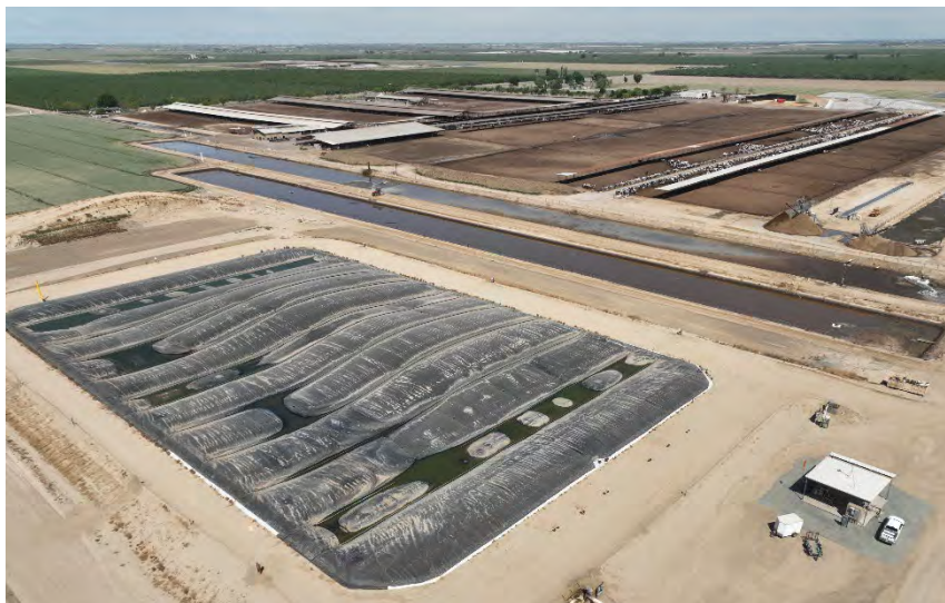
Image 76. New covered lagoon digester and conditioning skid at JR Dairy.
