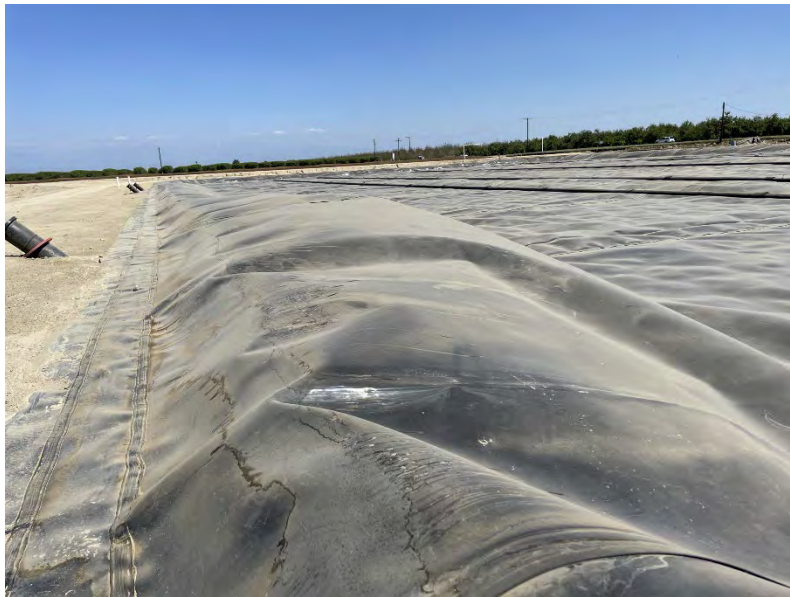
Image 45. Close up of the new covered lagoon digester at Rancho Sierra Dairy.
