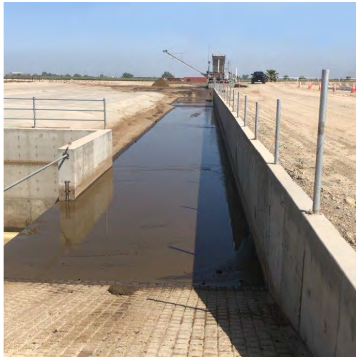
Image 49. New sand lane at El Monte Dairy.
