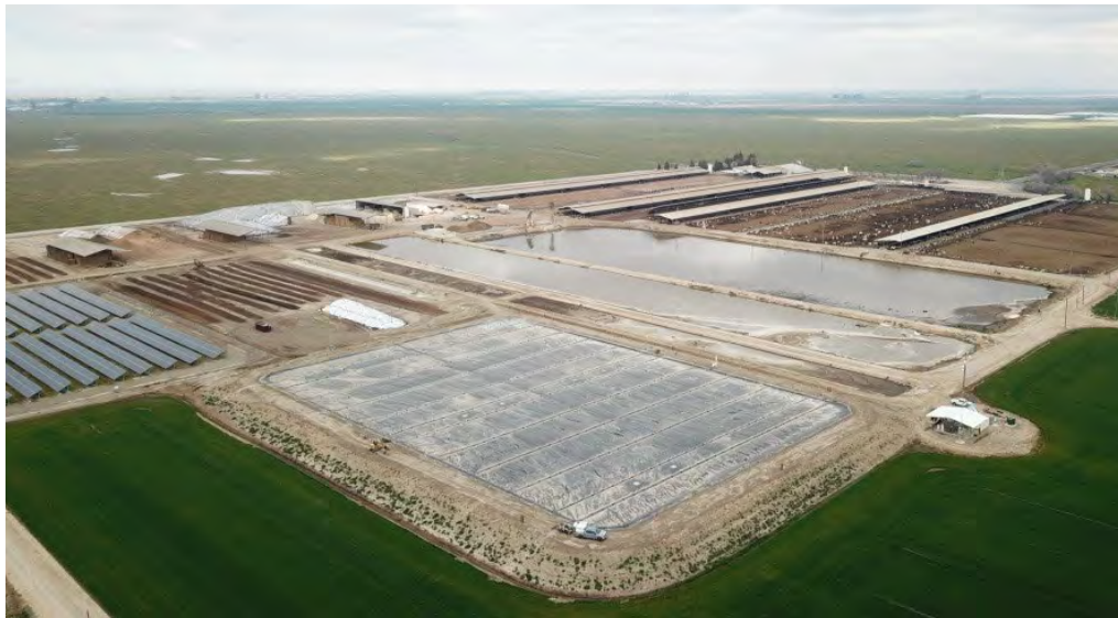
Image 75. New covered lagoon digester at Rockshar Dairy.
