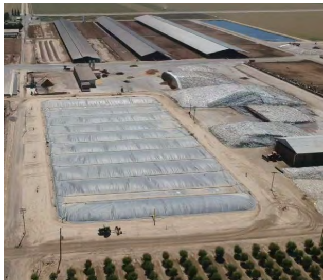
Image 74. New covered lagoon digester at Vista Verde Dairy.
