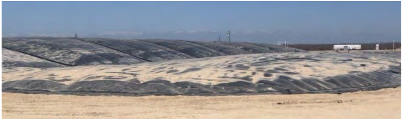
Image 36. Biogas build up in the new covered lagoon digester at Horizon Jerseys Dairy.
