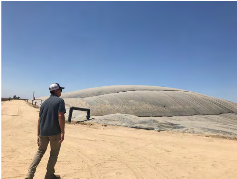
Image 13. Covered lagoon digester filled with biogas at the Vander Poel Dairy.
