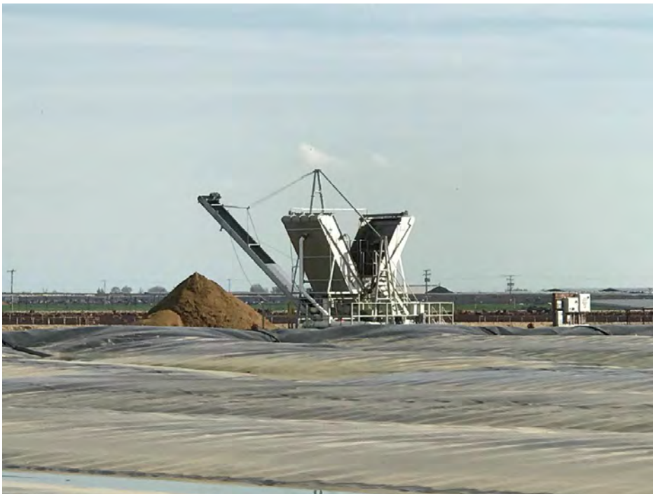
Image 10. Covered lagoon digester (foreground) and solid separator (background) at Legacy Dairy.
