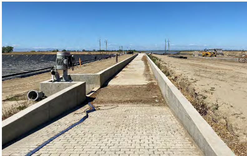
Image 63. New sand lane at Five H Dairy.
