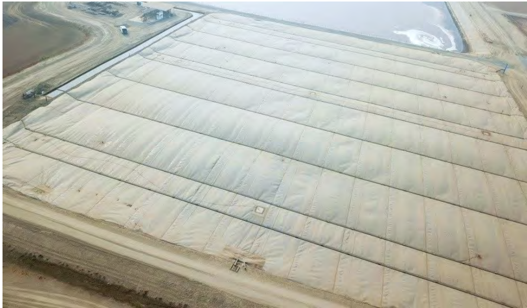
Image 51. New covered lagoon digester at Decade Dairy.
