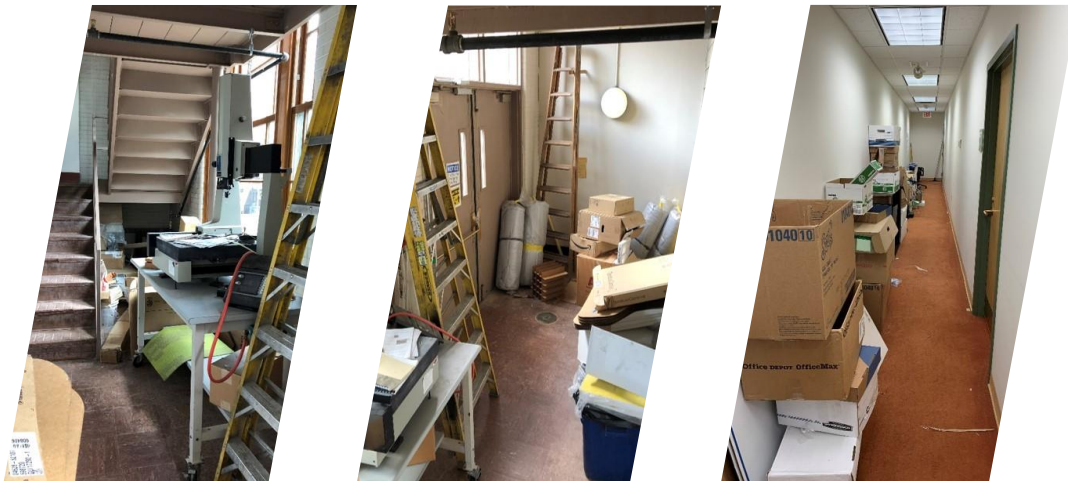
Examples of obstructed egress
