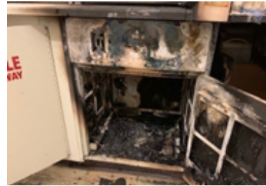
Image of the vacuum pump cabinet after the explosion from the University of Pennsylvania's EHR website
