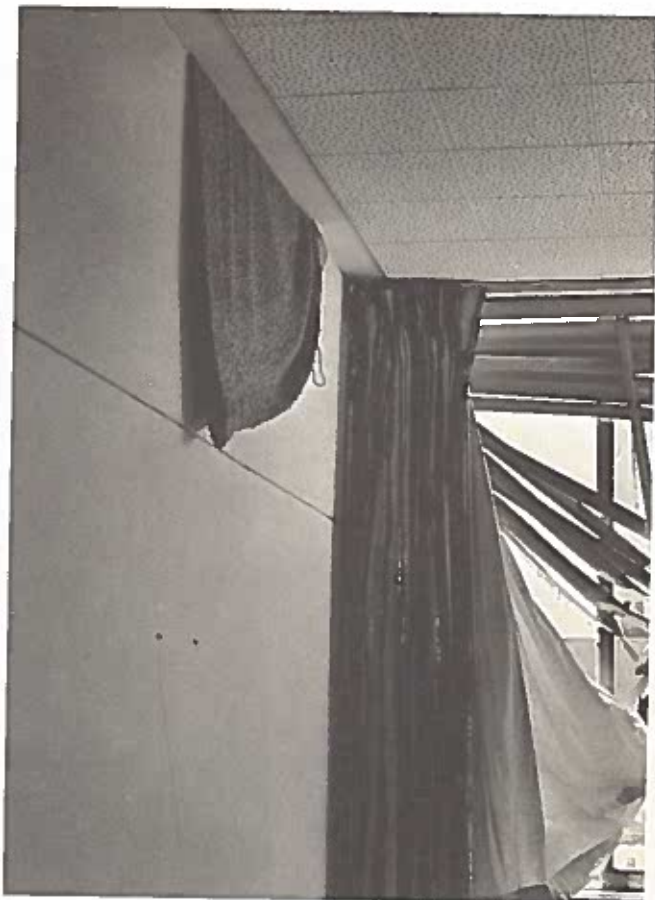
Draperies in Great Plains Life Building were blown into next office as force of the tornado separated ceiling from wall.
