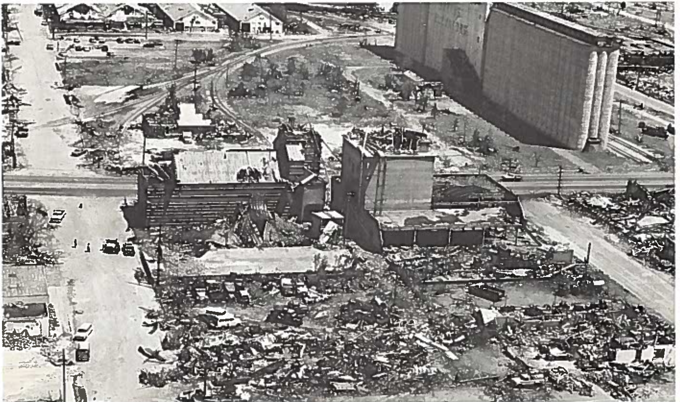
Storage elevators along 4th Street took a beating. One on the south side of street fell before the force of the winds.
