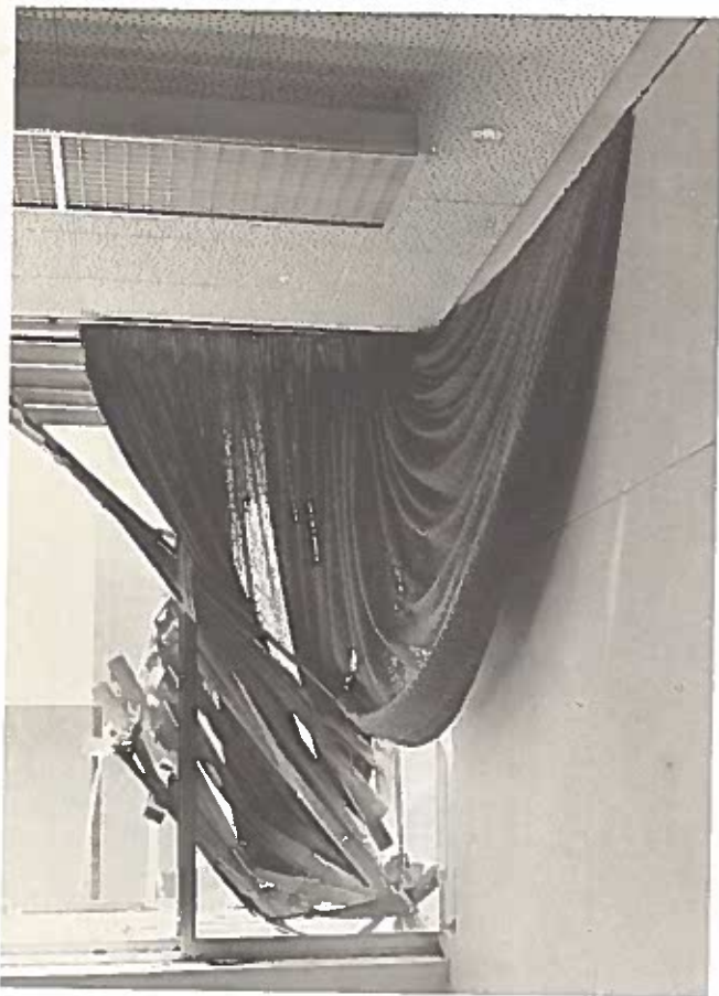
Draperies in Great Plains Life Building were blown into next office as force of the tornado separated ceiling from wall.
