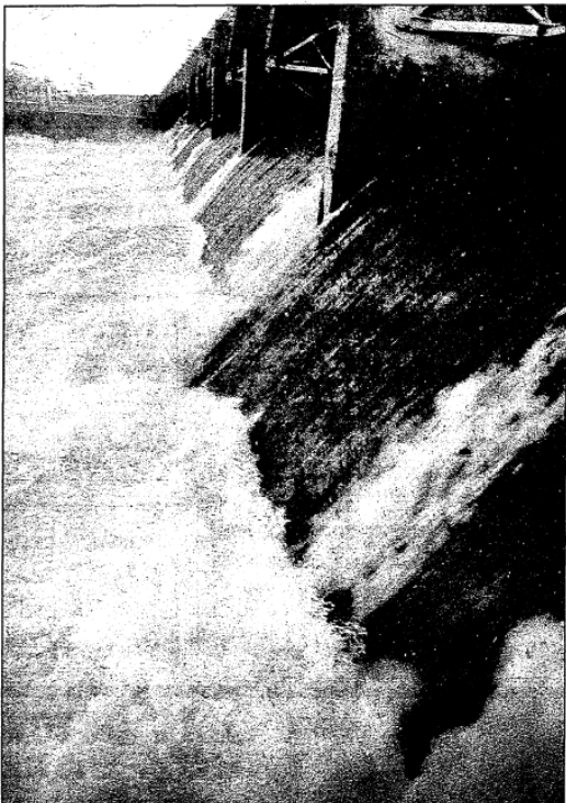
Water pours through the floodgates of the Santee Dam at a rate of almost 300,000 gallons per second Monday as Santee Cooper officials open the gates to eight feet to lessen the pressure on the dam from water flowing into Lake Marion. The water comes from rivers swollen from rain spawned by the remnants of Tropical Storm Marco. See story, Page 3-B.
