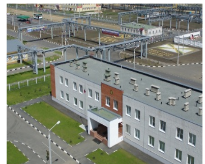
CW elimination and destruction facility in Russia
