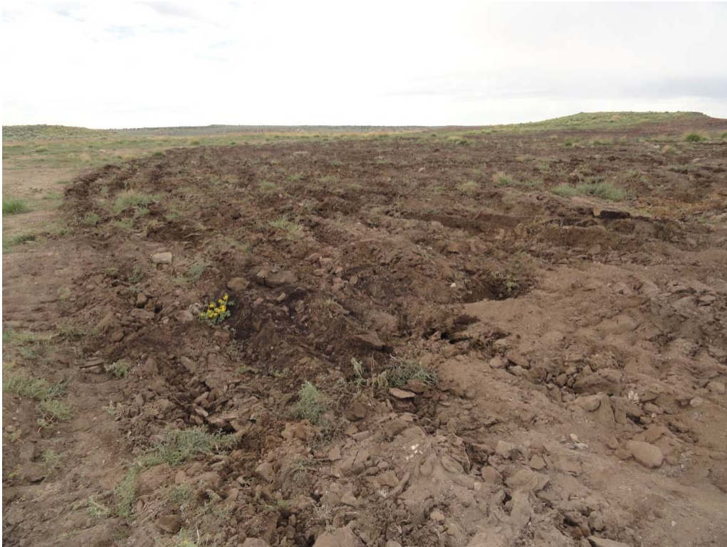
Deeply ripped mine reclamation in sandy, poorly developed soils
