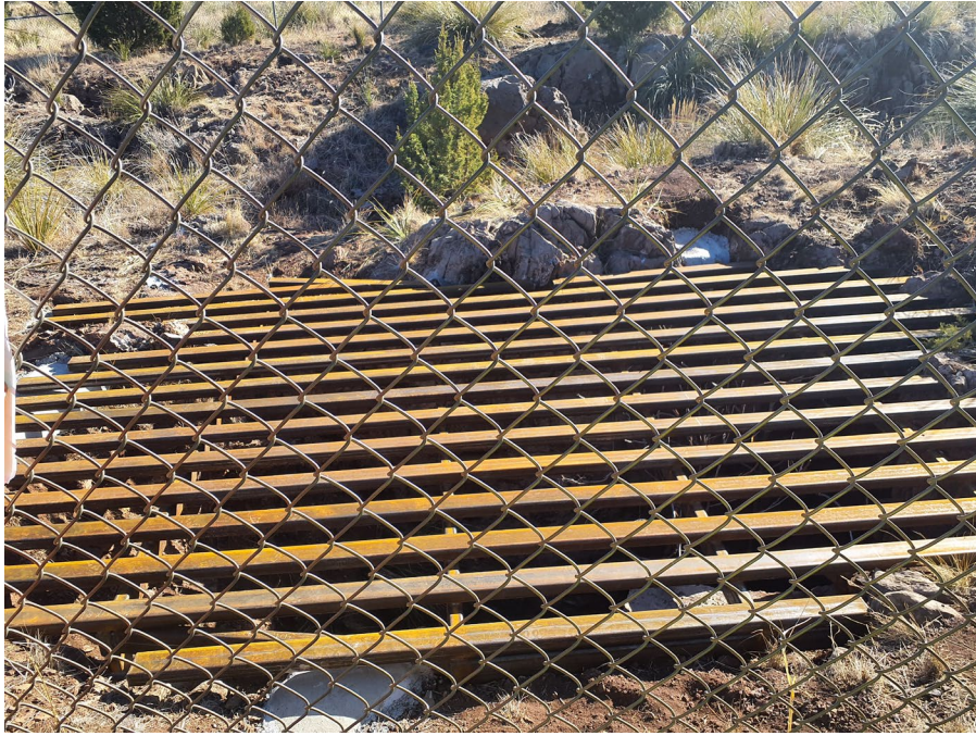
Figure 3: Open cut feature LT-140 with finished metal gate closure.
