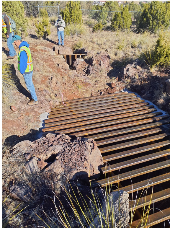
Figure 4: Open cut features LT-116 and LT-118 with finished metal gate closures.
