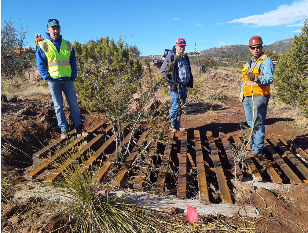
Figure 5: Open cut feature LT-115 with finished metal gate closure.
