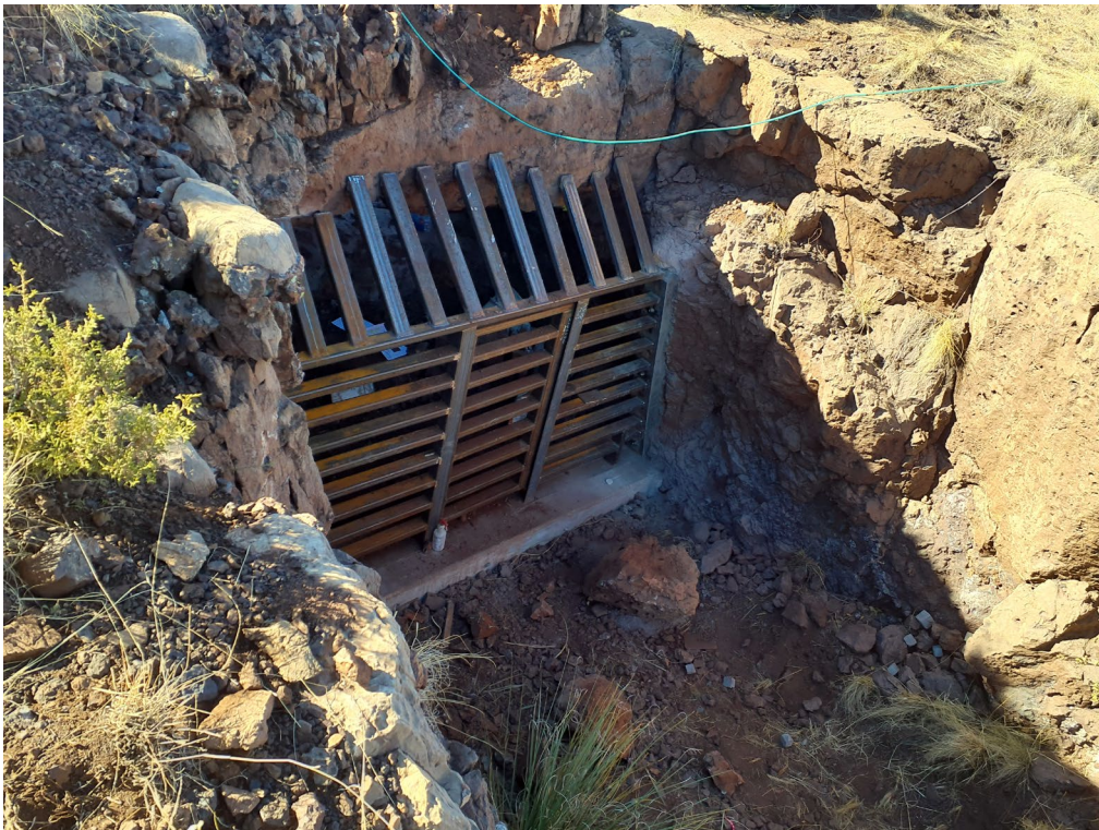
Figure 6: Adit feature LT-122 with finished metal gate closure.
