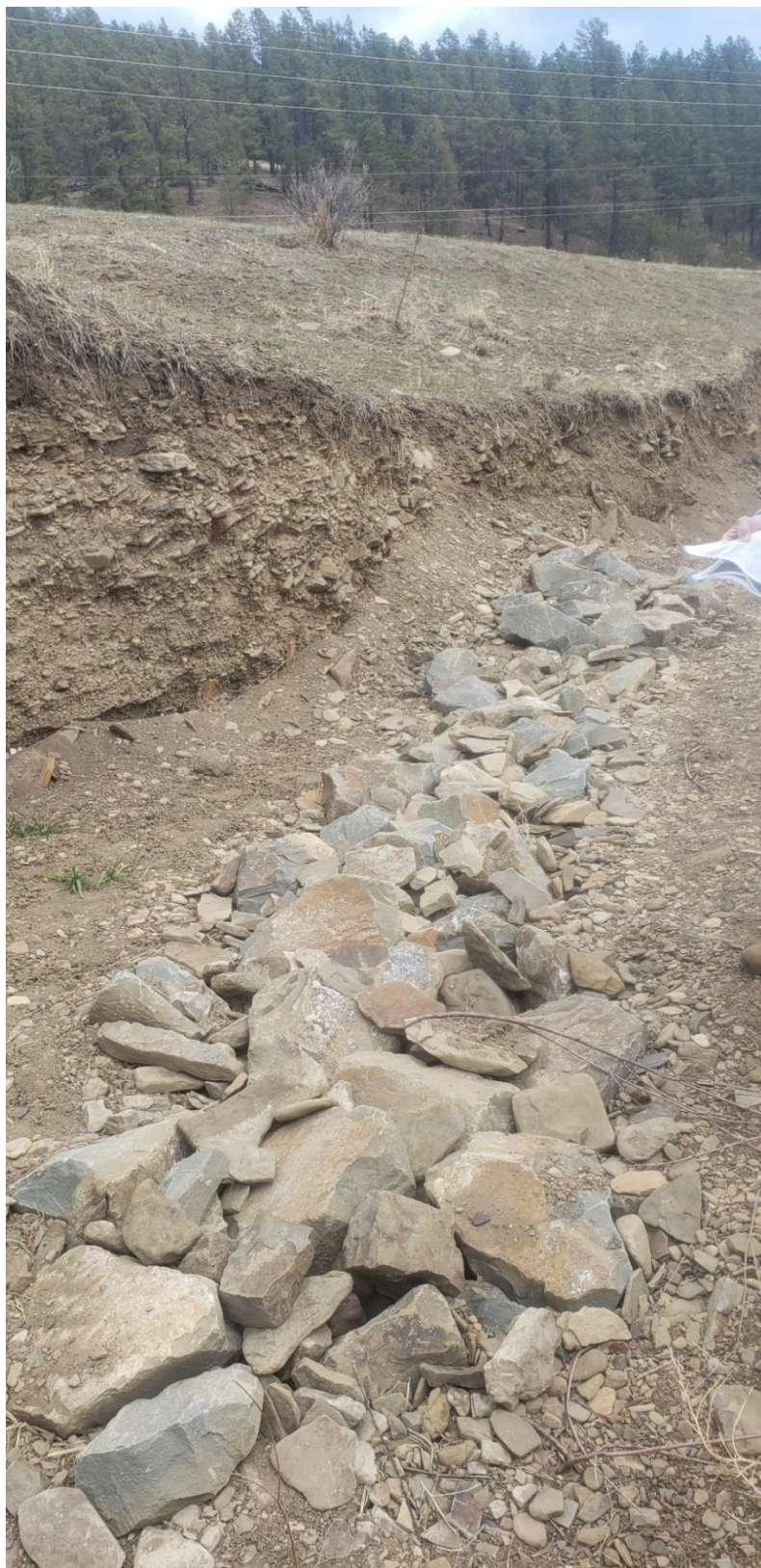
Figure 18. Rock armoring in Swastika Channel.
