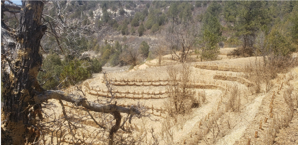
Figure 17. Coir roll and straw bale terracing with seedlings.
