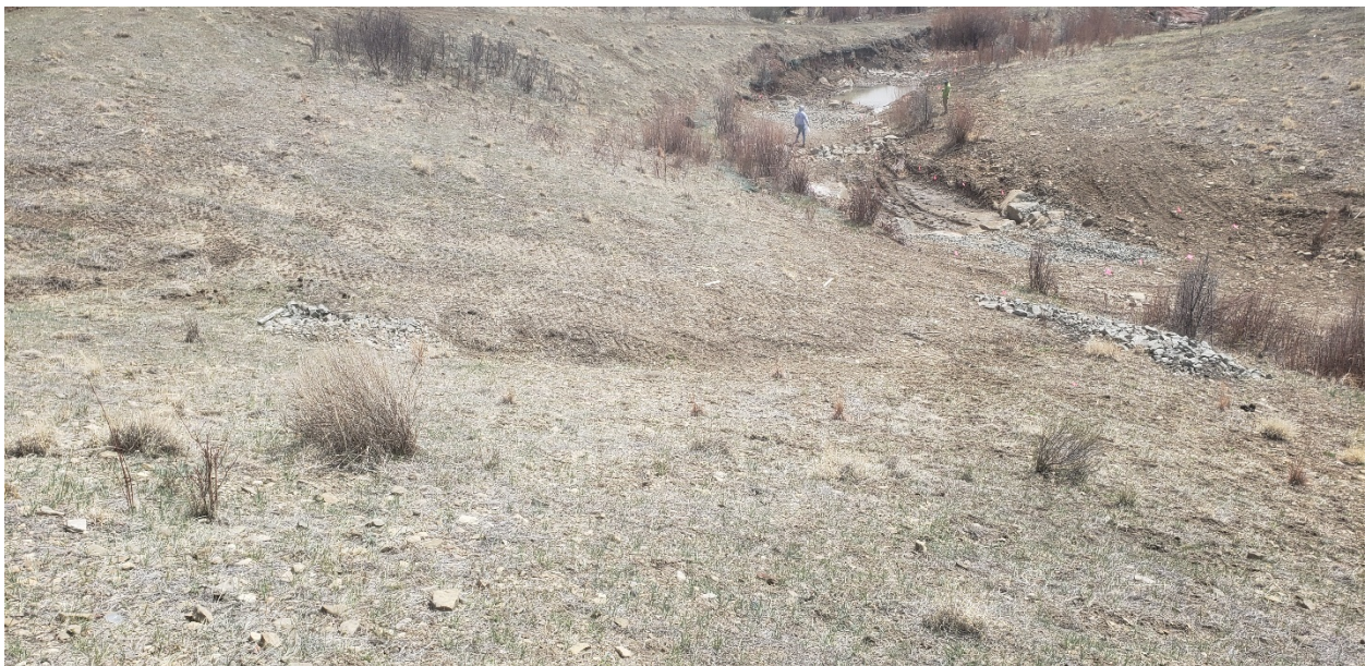
Figure 20. Channel sinuosity showcasing geomorphic design.
