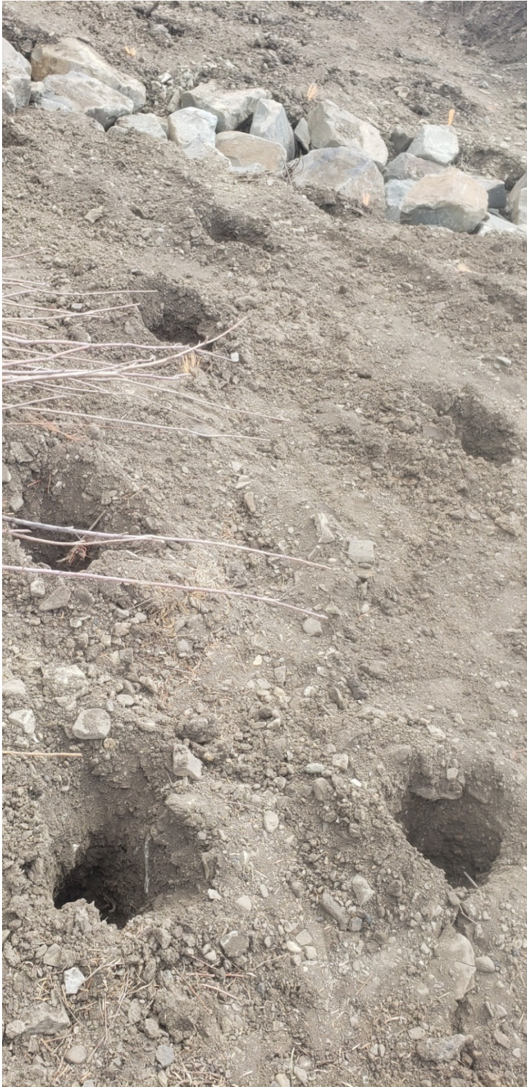
Figure 22. Augured holes in stream channel and embankment ready for willow and cottonwood plantings.
