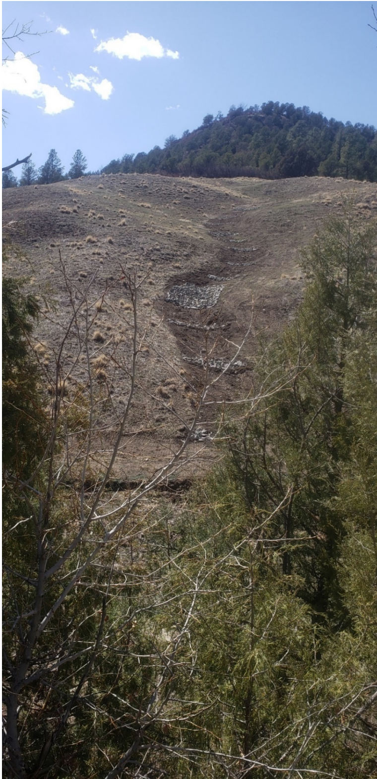
Figure 23. Geomorphic channel design and rock “medialuna” on reclaimed gob piles upland of Swastika Channel.
