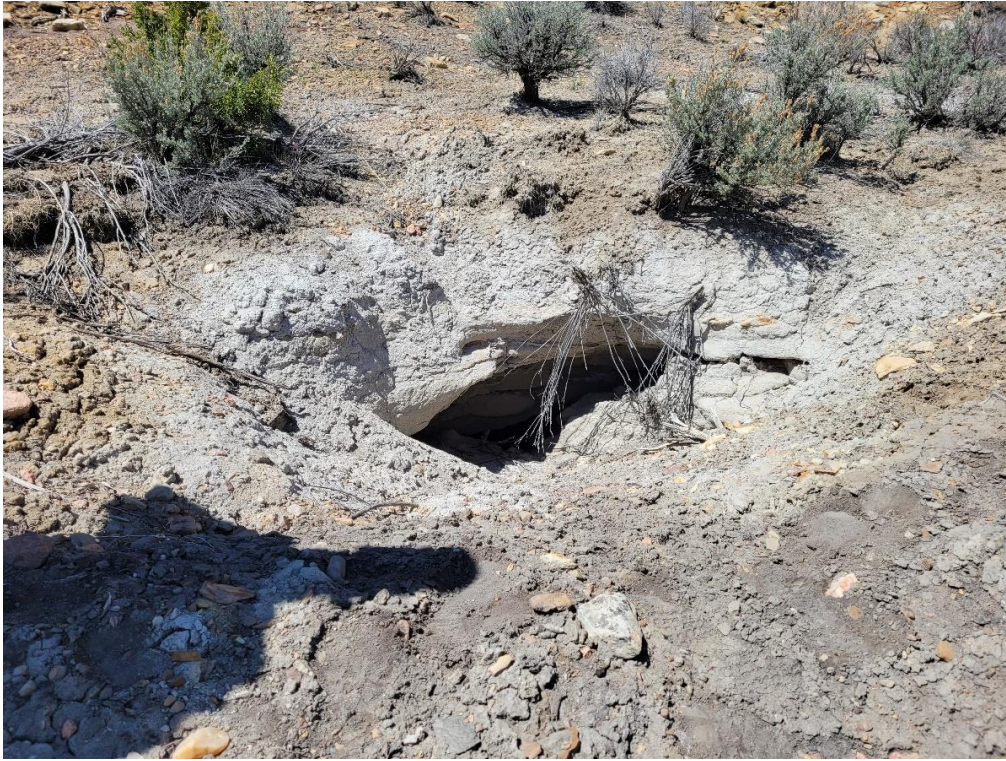
Figure 14: La Ventana Mine Closure Project, Kistler Black Rose Mine, Feature LV-6.
