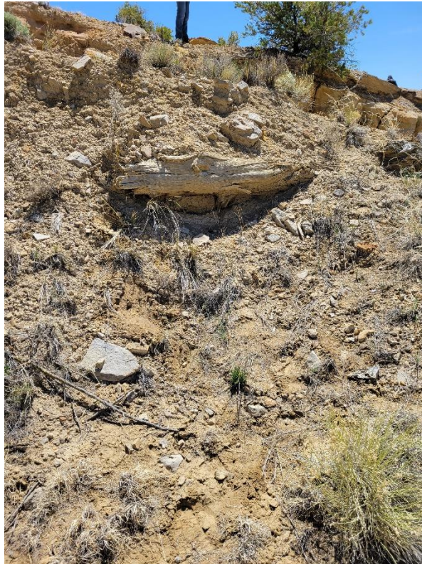
Figure 12: La Ventana Mine Closure Project, Kistler Black Rose Mine, Feature LV-3.
