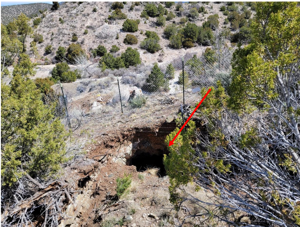
Figure 23: Harding Pegmatite Mine Safeguard Project, Sub-1 F
