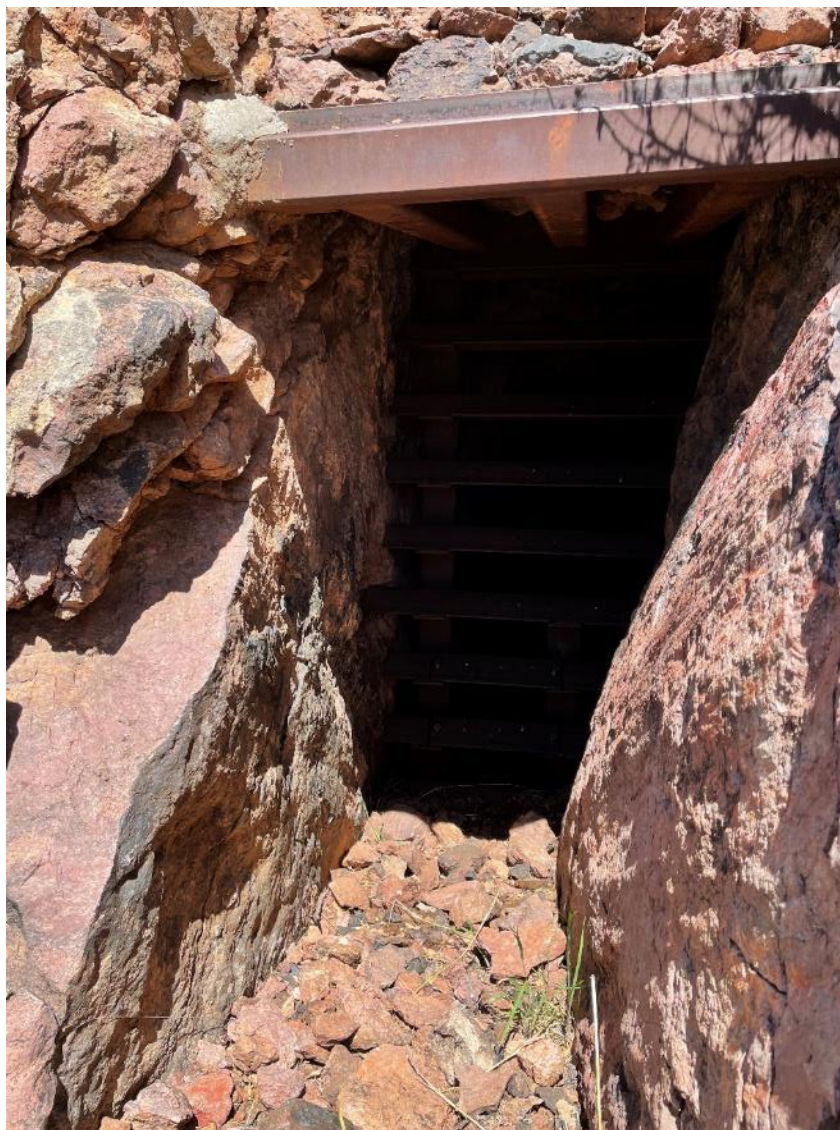
Figure 5: Socorro West Mine Safeguard Project, Nancy Mine, AML-4A.
