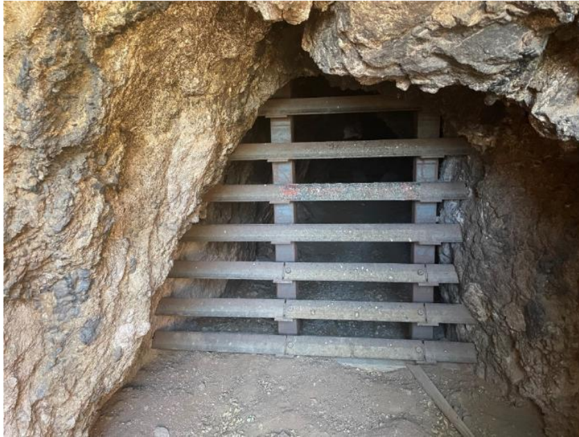
Figure 19: Socorro West Mine Safeguard Project, Black Canyon Mine, AML-7.
