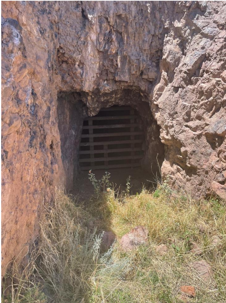
Figure 18: Socorro West Mine Safeguard Project, Black Canyon Mine, AML-6.
