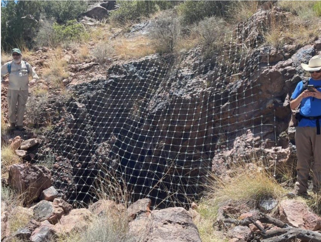
Figure 16: Socorro West Mine Safeguard Project, Black Canyon Mine, AML-6A.
