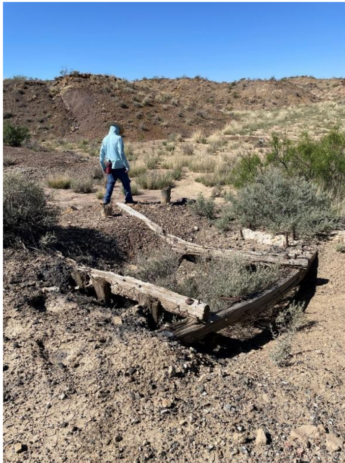
Figure 26: Carthage Mine Safeguard Project, Government and Duffy Mines, C-3.
