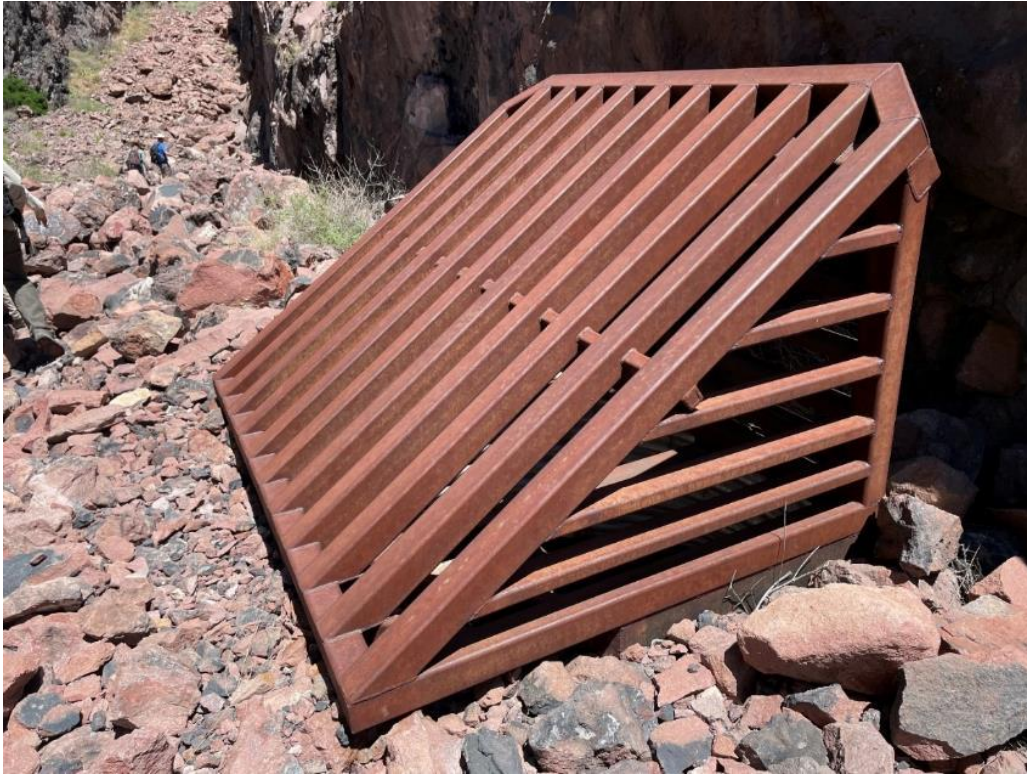
Figure 10: Socorro West Mine Safeguard Project, Nancy Mine, AML-13.
