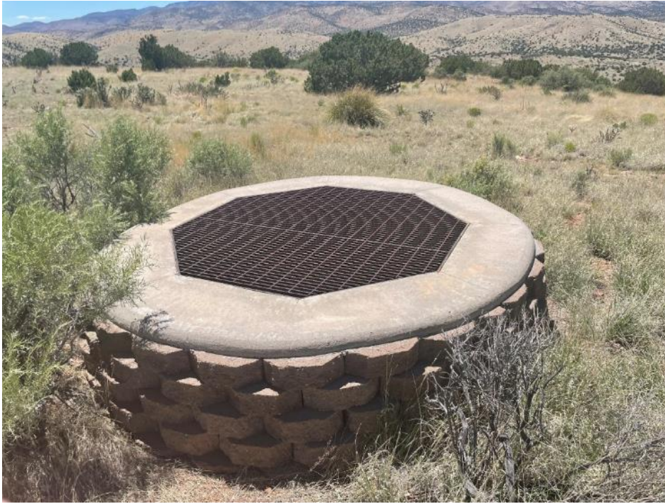
Figure 21: Socorro West Mine Safeguard Project, Black Canyon Mine, AML-11.
