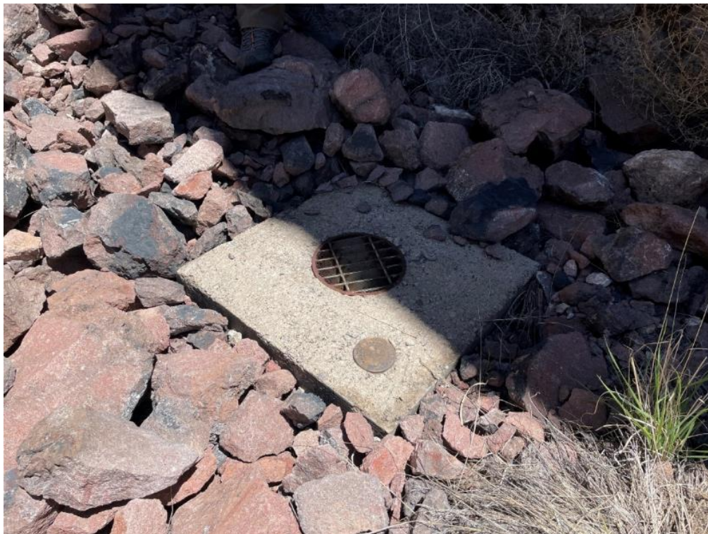
Figure 11: Socorro West Mine Safeguard Project, Nancy Mine, AML-13.5.
