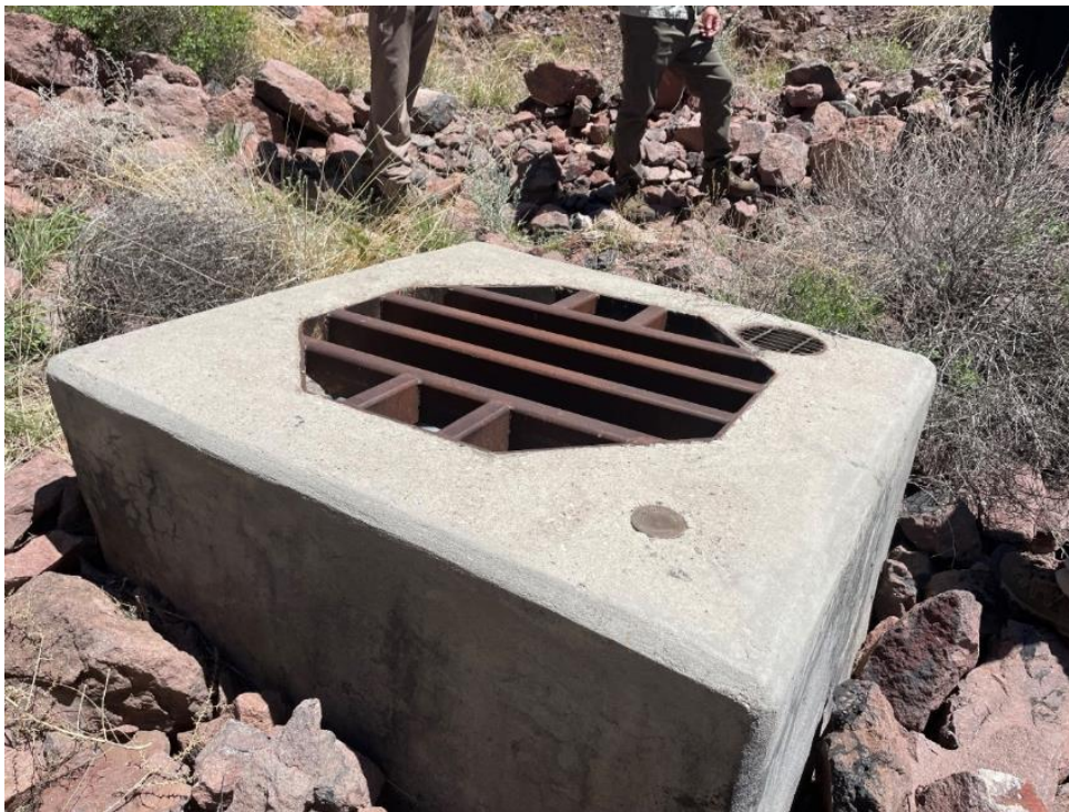
Figure 13: Socorro West Mine Safeguard Project, Nancy Mine, AML-17.
