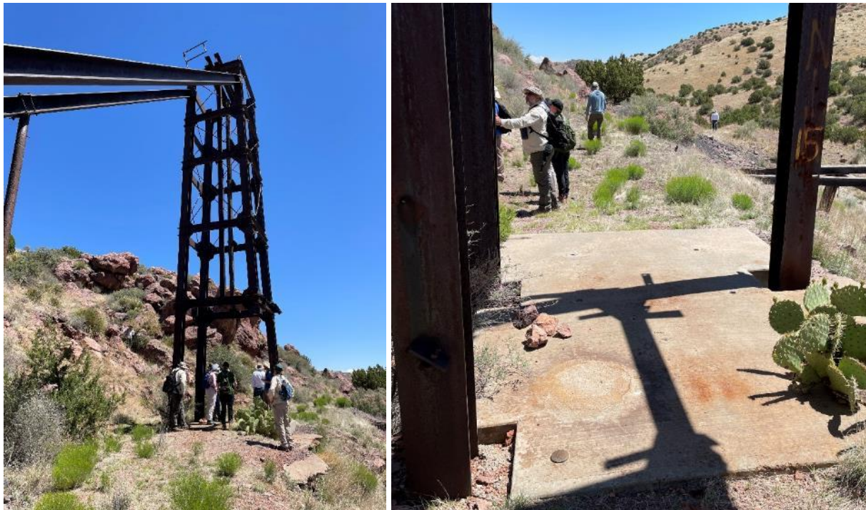
Figure 4: Socorro West Mine Safeguard Project, Nancy Mine, AML-4.
