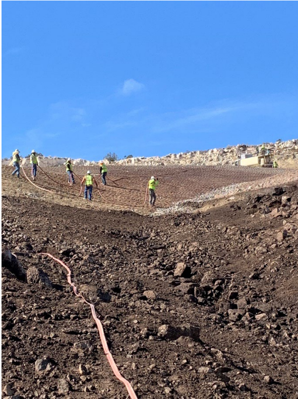
Hydroseeding at Tijeras Mine
