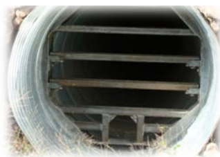
Figure 4 Culvert with Bat gate
