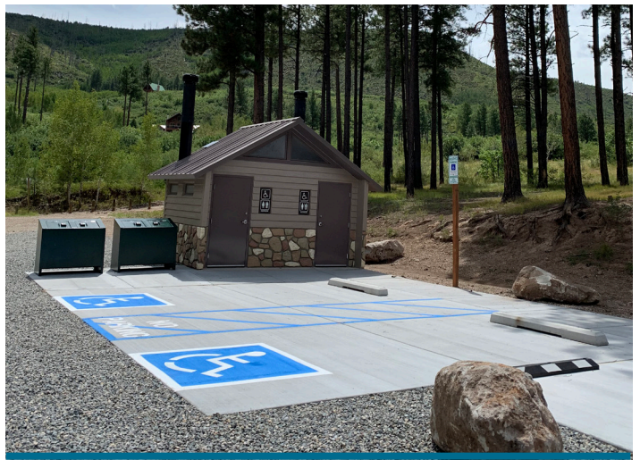
Double vault toilet with Americans with Disabilities Act (ADA) approved parking & trash receptacles
