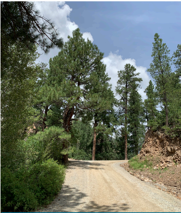
Lake Fork Road Improvements Looking North
