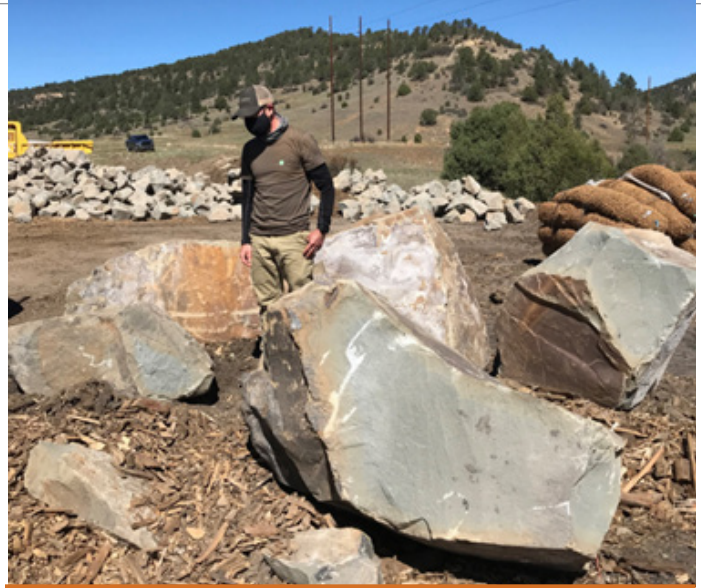
Large boulders were brought in as part of the design structures to slow the water down.
