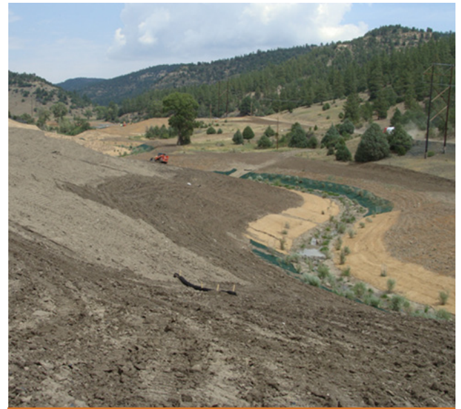
2012 photo shows the stream recontoured into a winding route, and the buried gob and clean soil cap contoured into a geomorphic surface that blended in with the natural topography.
