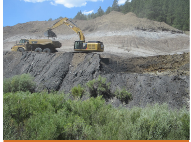
Heavy equipment at Dutchman Canyon coal mine burying the gob pile near the stream channel
