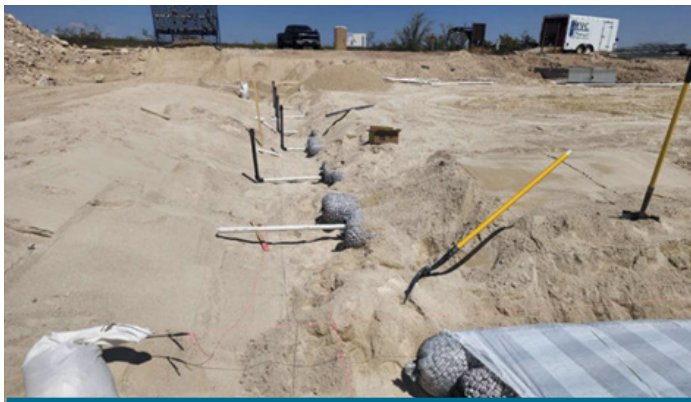
Evapotranspiration Bed end view of distribution bundles
