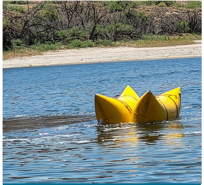
Removal of car from Lazy Lagoon sinkhole at Bottomless Lakes State Park by tying floats to it to raise it 60 feet to the surface.
