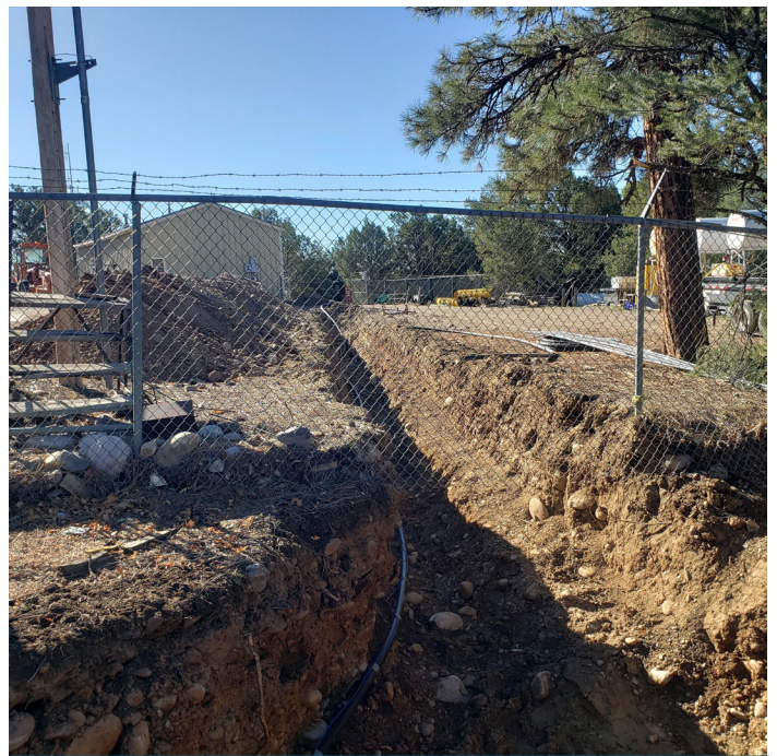
Heron Lake Water Treatment Plant in background
