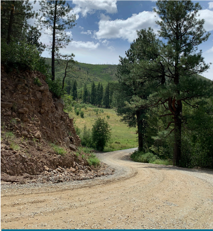
Lake Fork Road Improvements Looking South
