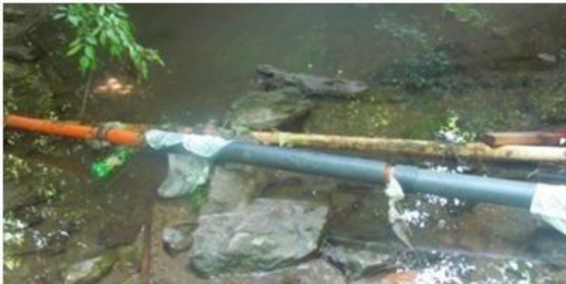
Figure 37. Utility line crossing stream
