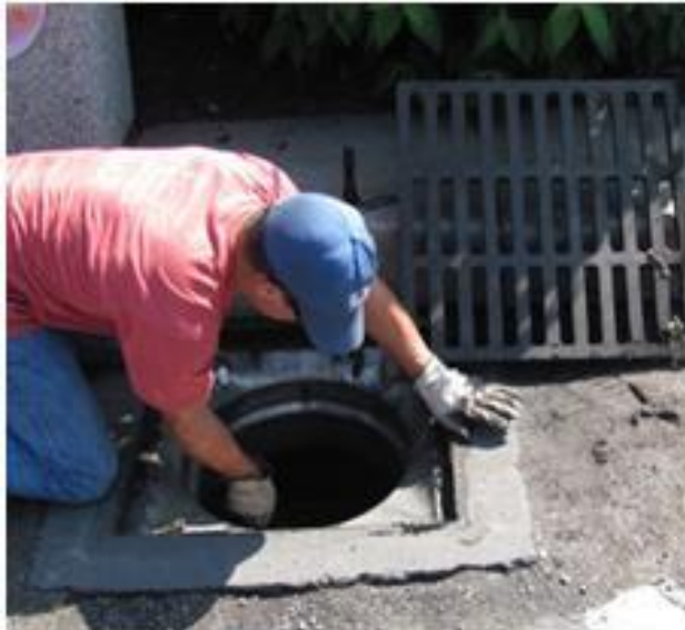
Figure 45. Source of foul odor
