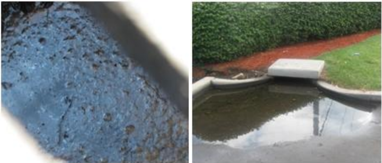
Figure 46. Water with sheen and brown foam; Water pooling around drain
