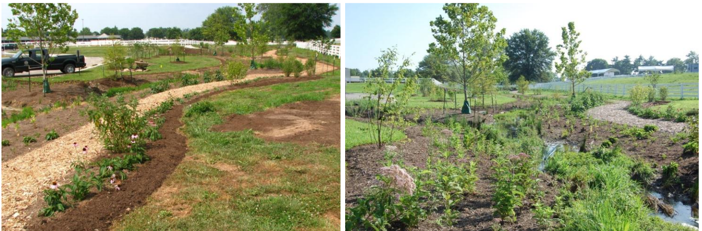
Figure 150. The streamside vegetated buffer along a tributary of the Cane Run under construction and completed
