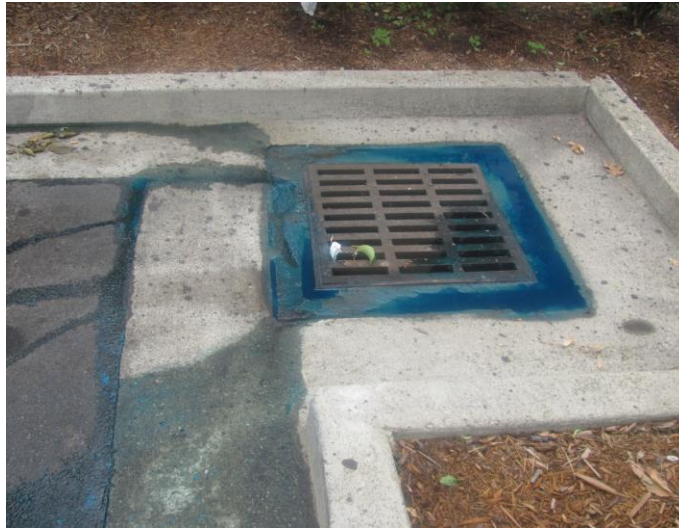
Figure 48. Blue substance entering drain
