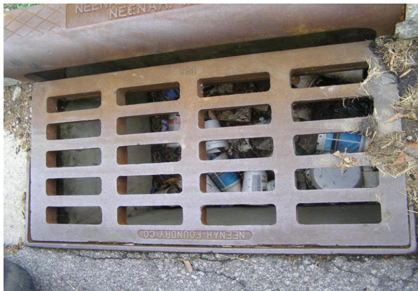
Figure 51. Trash-filled drain
