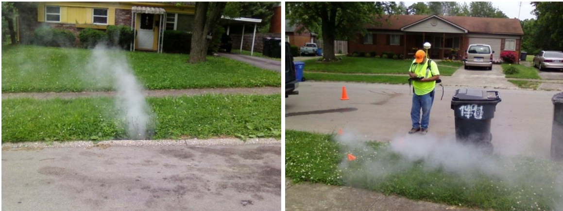
Figure 84. LFUCG sanitary sewer smoke testing coming out of storm sewer
