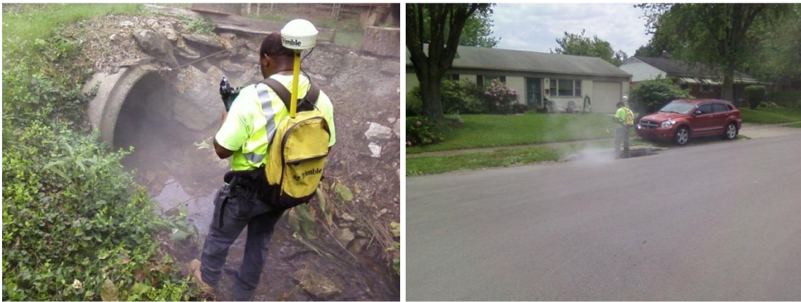
Figure 83. LFUCG sanitary sewer smoke testing coming out of storm sewer
