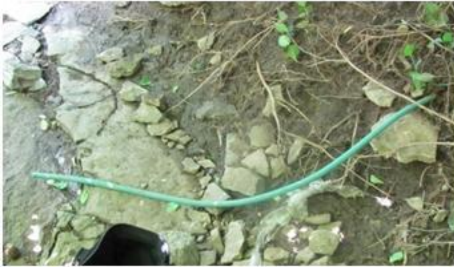
Figure 34. Garden hose sticking out of side of bank
