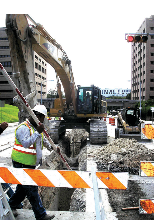
Construction of city-supplied reclaimed water distribution lines
