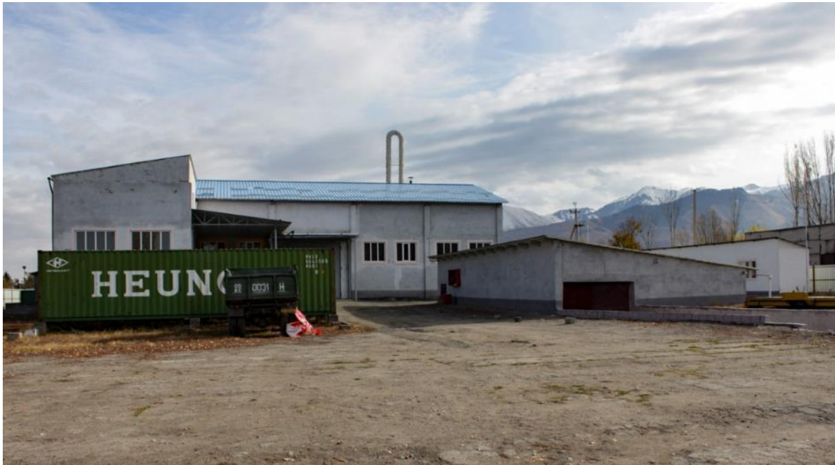
Figure 9. Non-functioning starch factory – a view from outside
