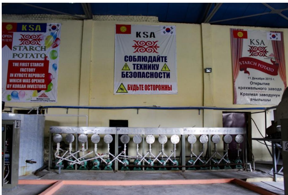
Figure 10. Non-functioning starch factory – a view from inside
