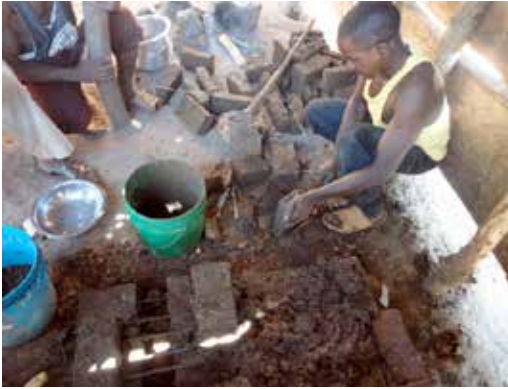
Figure 3: Preparing the basement for the improved stove
