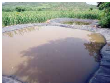
Figure 4: Rainwater harvesting ponds lined with geo-membrane
