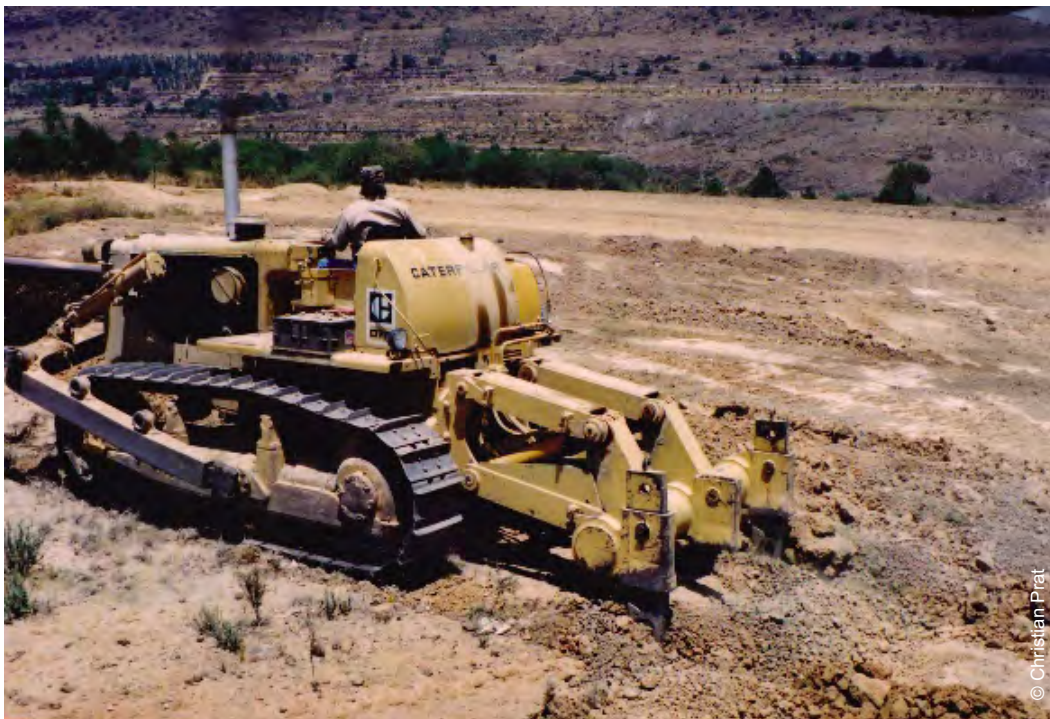
Photo 79. Heavy machinery breaking
