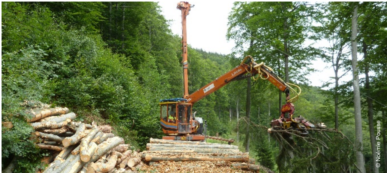
Photo 1. Soil disturbance (rut formation and soil compaction) from conventional skidder logging in Austria (top left) and France (top right). Cable yarding operation in the Austrian Alps (bottom)
