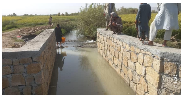
Completed Turkman Drainage in Faryab Province.
