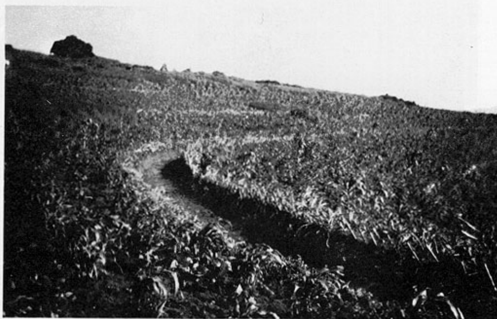
FIGURE 48. - Example of diversion channel with other soil conservation practice, in this case trash bunding. The bank is planted with Napier grass ( Pennisetum purpureum ) to strengthen it and to provide fodder. (Tanzania: Photo by I. Constantinesco)
