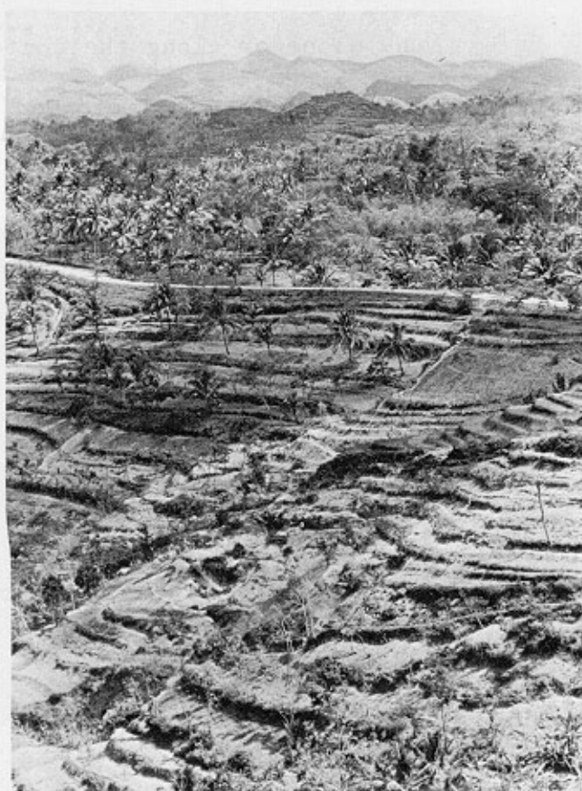
FIGURE 53. - Breakdown of terrace banks due to poor design and lack of maintenance in Java, Indonesia. (FAO photo by H. Hull)
