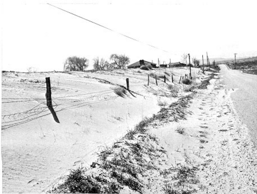
FIGURE 16. - Result of wind erosion. The borrow pit has been completely filled, soil has drifted onto the road and against the fence, destroying it in the process. (Idaho, U.S.A. Photo courtesy of USDA Soil Conservation Service)
