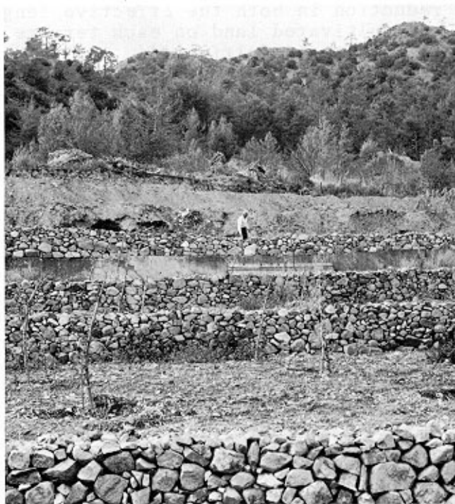
FIGURE 50. - Stone-wall bench terraces in the Troodos mountain region in Cyprus. (FAO Photo by J. Ciganovic)
