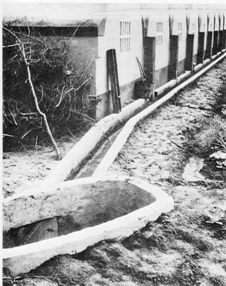
Fig. 33 Building of piggery with inlet for animal wastes to bio-gas plant. Cheng Hsiang Production Brigade, Jiangsu Province.
