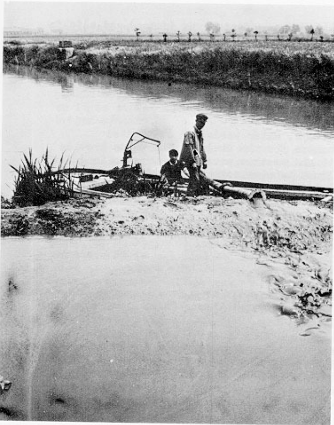
Fig. 6 Boat for sucking silt from the bottom of the canal. Foreground: Silt tank. Malu People's Commune, Shanghai
