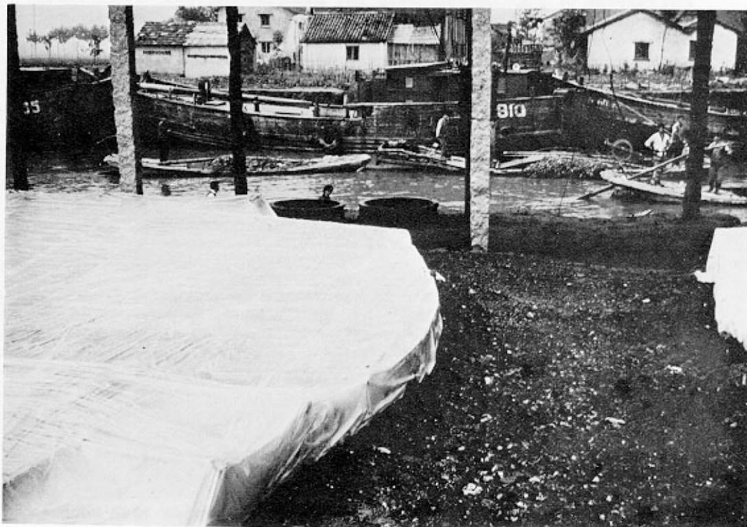
Fig. 3 Foreground: Concrete tanks for night soil covered with plastic. Background: Transport of garbage from Shanghai. Malu People's Commune, Shanghai.
