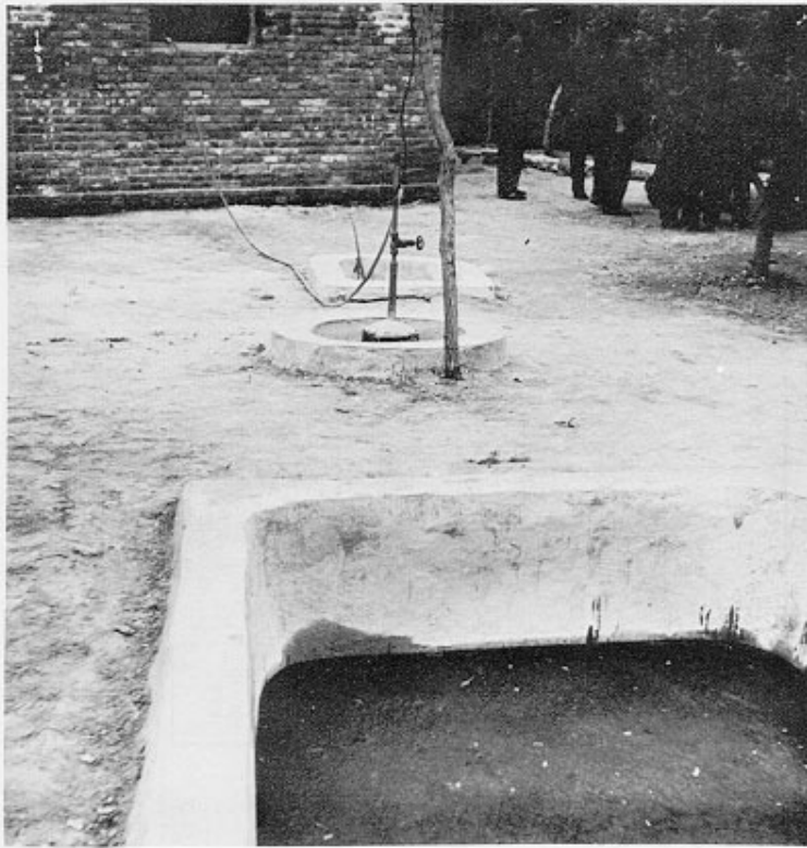
Fig. 45 Larger size bio-gas plant, gas used to fuel diesel engine. Foreground: outlet; centre: outlet for gas by plastic pipe; background: inlet. Chun Sun Production Brigade, Hebei Province.
