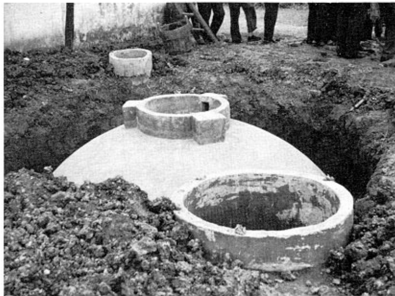
Plate 23. The biogas unit shown under construction in Plates 21 and 22, after its initial plastering. The outlet is in the foreground and the inlet in the background.
