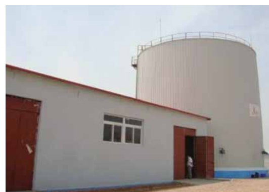
FIGURE 6.16 Biogas fermentation and biogas capture tank using straw fermentation on an industrial scale in Jinghai, Tianjin.
