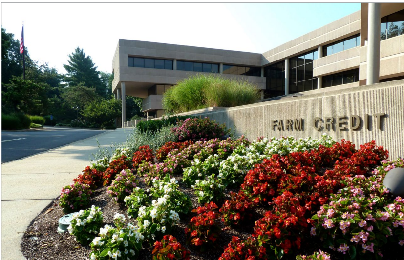
The headquarters of the Farm Credit Administration, located in McLean, Virginia.
