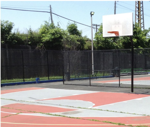
Figure A3: NYCHA South Jamaica Houses cloudburst pilot. The existing basketball court will be excavated to create underground water storage and repair the surface. The new "cloudburst" design will lower the basketball court, allowing it to fill with water during extreme rain, and providing a new seating area for residents
