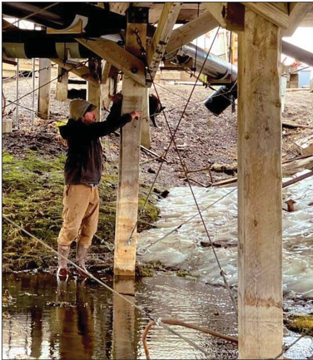
Figure 5. Assessing subsidence below homes in Point Lay. Melting ice wedges below this home have resulted in nearly 2 m (6.5 ft) of subsidence leaving only about 1 m (3.2 ft) of pile embedment. (Credit: P. Bolz)
